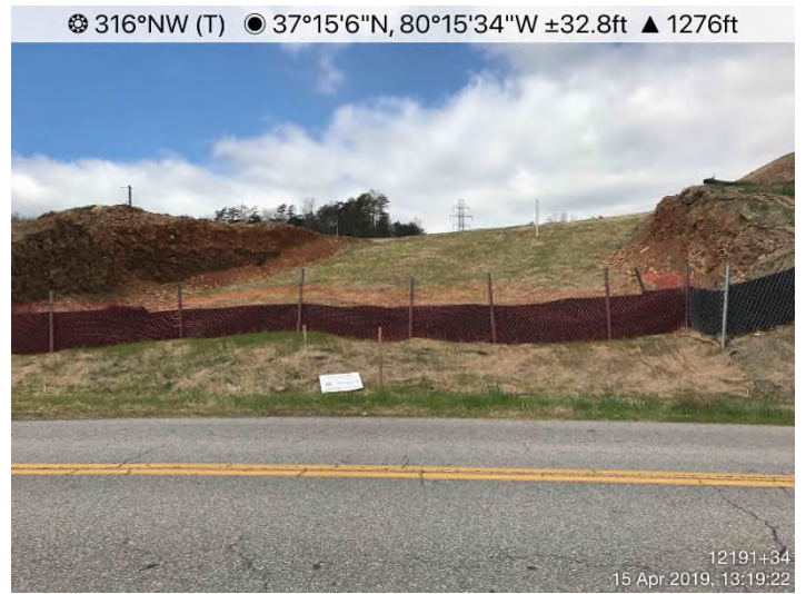
Fig. 4: STA 12191+34 – Area adequately stabilized. Controls in place.
