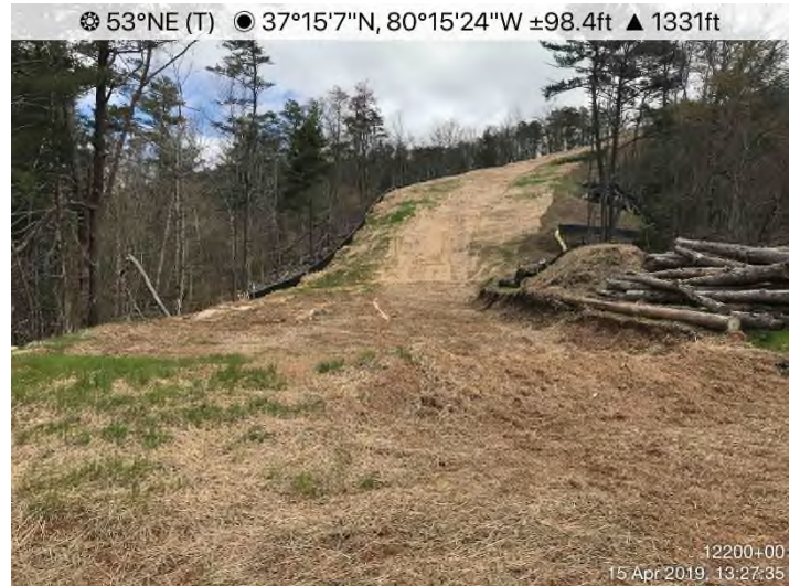
Fig. 8: STA 12207+99 – Area adequately stabilized. Controls in place.
