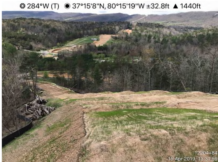
Fig. 7: STA 12204+84 – Area adequately stabilized. Controls in place.
