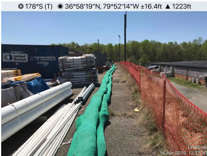
Fig. 3: LY 045/046 – Perimeter controls in place.
