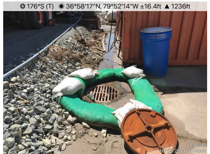
Fig. 4: LY 045/046 – Inlet protection in place.
