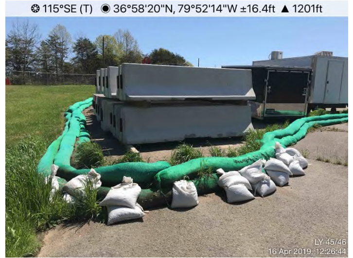
Fig. 4: LY 045/046 – Inlet protection in place.
