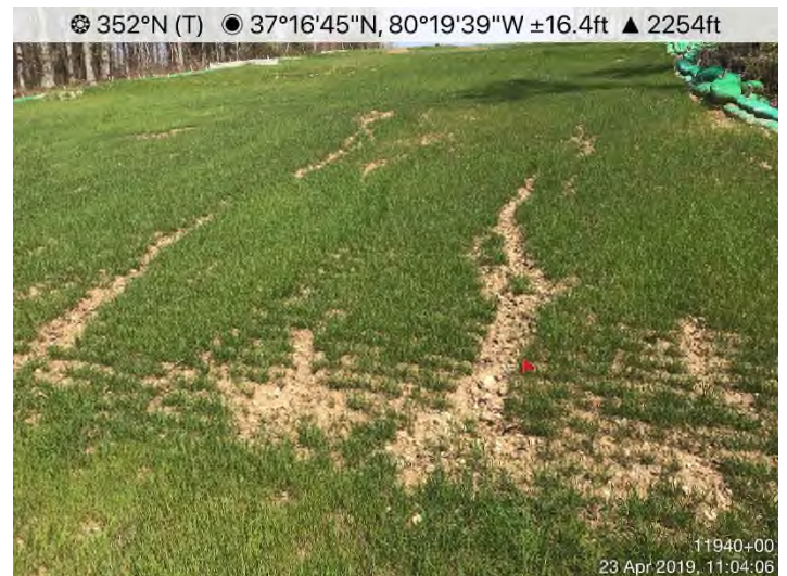
Fig. 4: STA 11940+00 – Rill erosion occurring.
