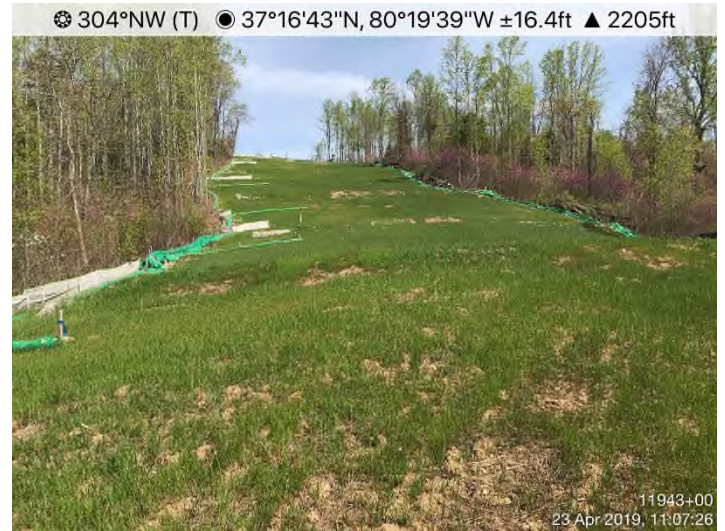
Fig. 4: STA 11940+00 – Rill erosion occurring.
