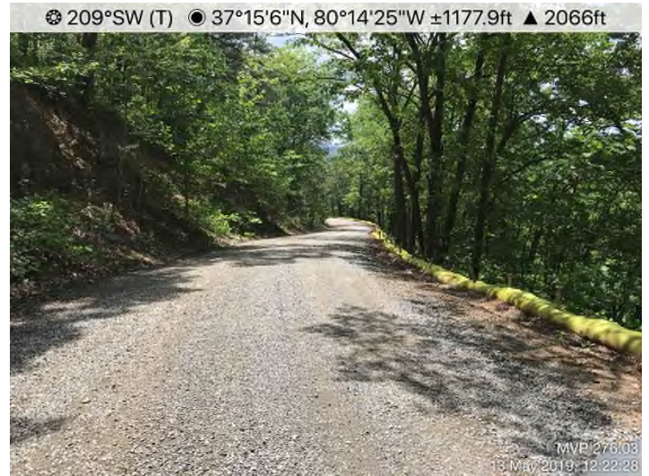
Fig. 4: PY-006 – Secondary containment controls in place.
