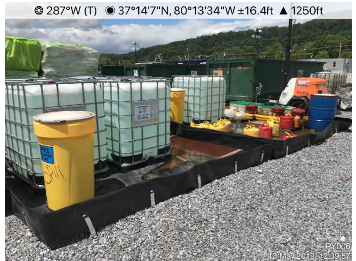
Fig. 4: PY-006 – Secondary containment controls in place.
