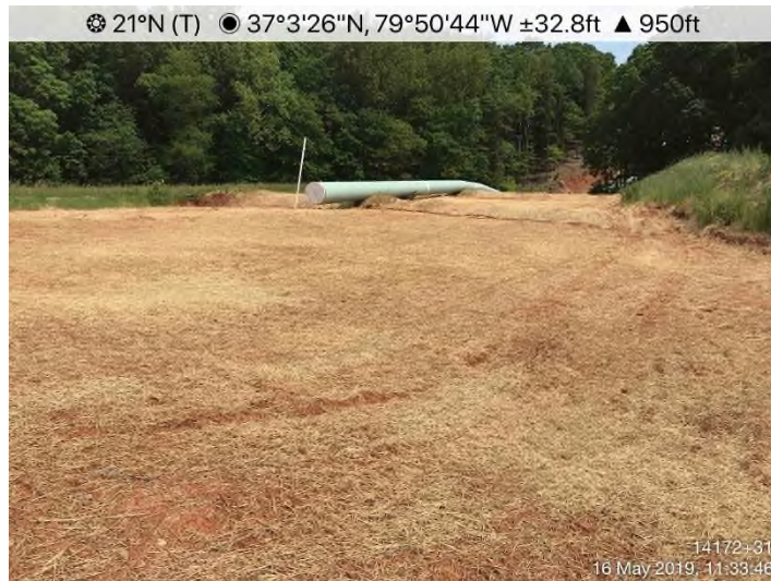
Fig. 7: STA 14185+00 – Area stabilized with straw. Controls in place.
