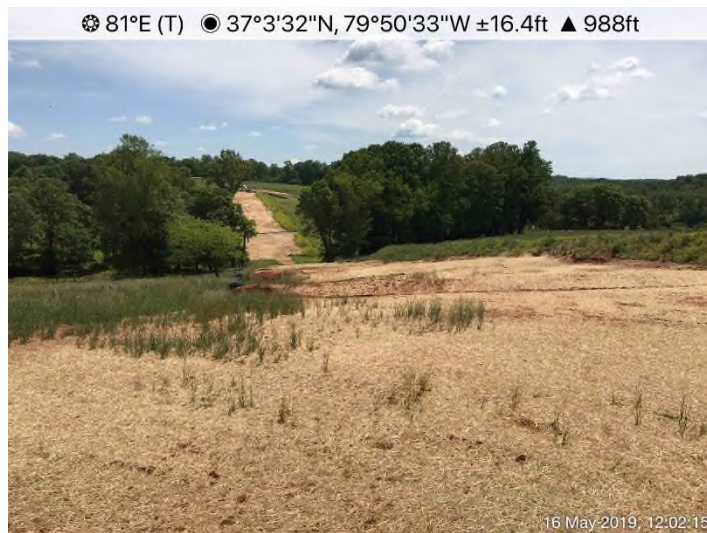
Fig. 7: STA 14185+00 – Area stabilized with straw. Controls in place.
