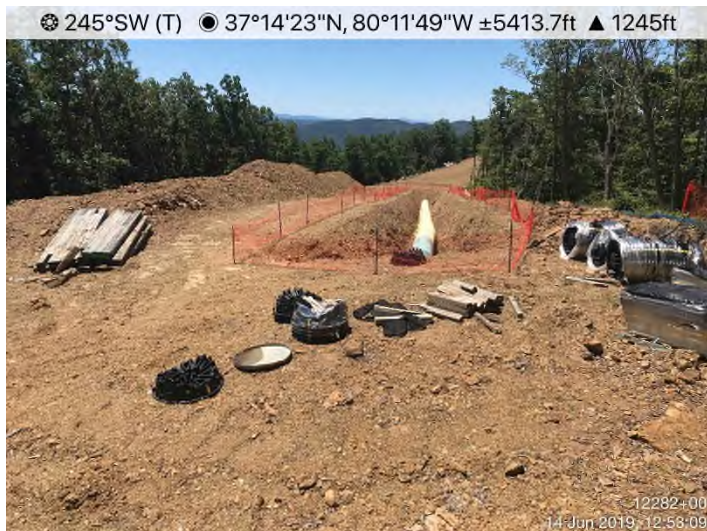
Fig. 3: STA 121282 – Controls in place. Area stabilized with Earth-Guard.
