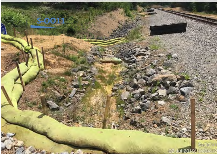
Fig. 11: Photo Location "K" – Sediment discharge from east side of Norfolk Southern ROW into Stream S-OO11.
