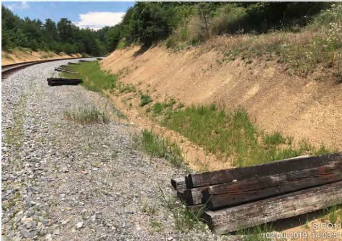
Fig. 11: Photo Location "K" – Sediment discharge from east side of Norfolk Southern ROW into Stream S-OO11.
