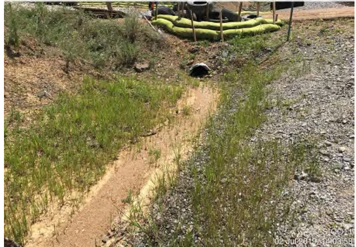
Fig. 12: Photo Location "L" – Sediment discharge from east side of Norfolk Southern ROW towards Stream S-OO11.
