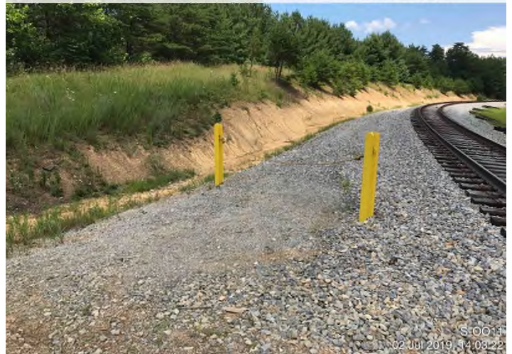
Fig. 8: Photo Location "H" – Denuded area on west side of Norfolk Southern ROW. Sediment is being discharged towards stream S-OO11.
