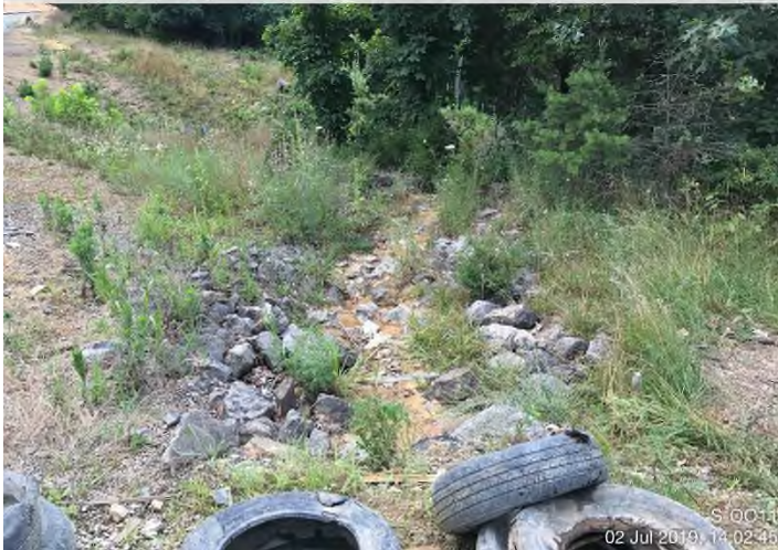
Fig. 7: Photo Location "G" – Sediment discharge from west side of Norfolk Southern ROW towards Stream S-OO11.
