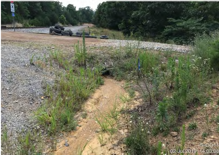
Fig. 7: Photo Location "G" – Sediment discharge from west side of Norfolk Southern ROW towards Stream S-OO11.
