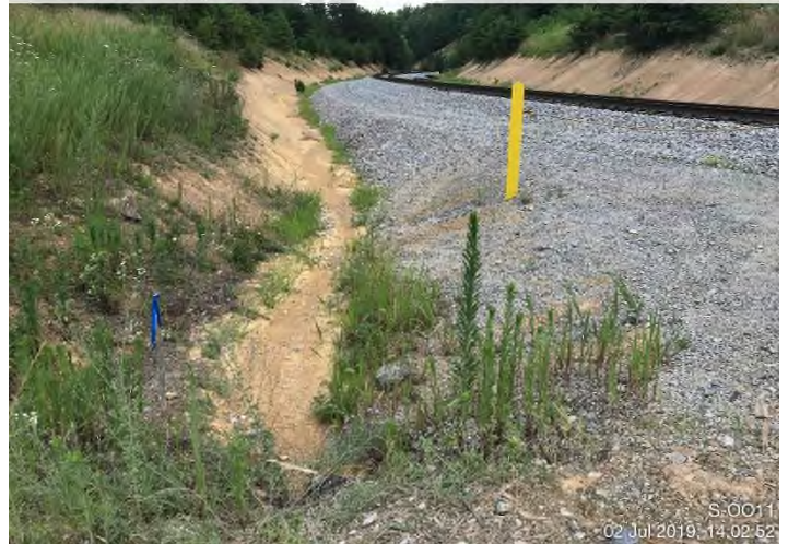
Fig. 8: Photo Location "H" – Denuded area on west side of Norfolk Southern ROW. Sediment is being discharged towards stream S-OO11.
