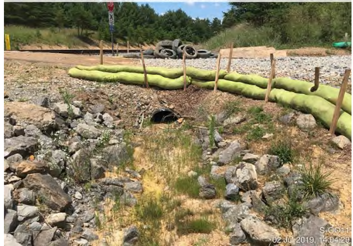
Fig. 12: Photo Location "L" – Sediment discharge from east side of Norfolk Southern ROW towards Stream S-OO11.
