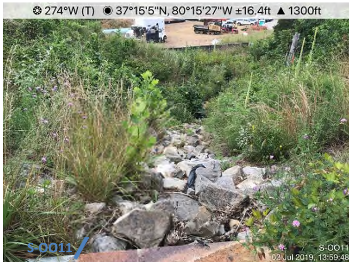
Fig. 3: Photo Location "C" – Sediment discharge from west side of Norfolk Southern ROW towards Stream S-0011.
