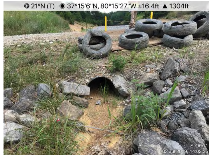
Fig. 4: Photo Location "D" – Sediment discharge from west side of Norfolk Southern ROW towards Stream S-0011.
