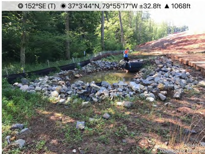
Fig. 3: STA 13844+07 to 13846+78 – Repair and stabilize perimeter berms.
