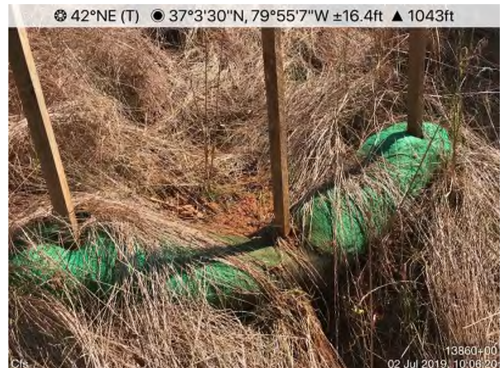
Fig. 4: STA 13860+00 – CFS maintenance needed.
