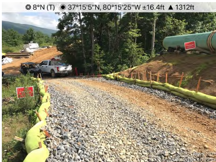
Fig. 11: ATWS 1375 – Looking north from ATWS 1375 towards stream S-OO11. CFS is in good condition. Dormant areas stabilized with seed, straw and fabric.
