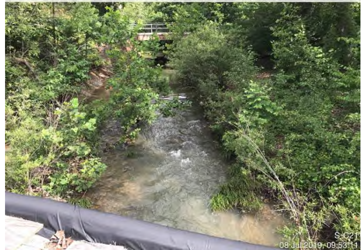
Fig. 4: ATWS 704A – Perimeter controls adjacent to S-C21 (Bradshaw Creek). SSF installed correctly and functioning properly. Dormant storage area within LOD stabilized with seed and straw.
