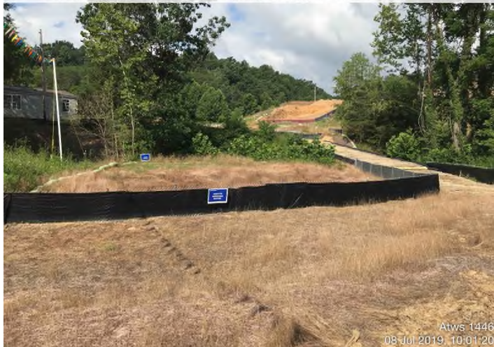
Fig. 7: Stream S-0011 – Sediment impacting S-0011 (UNT to Bradshaw Creek) at approx. STA 12196+24.
