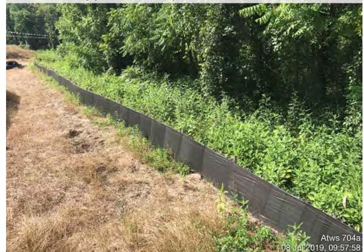
Fig. 4: ATWS 704A – Perimeter controls adjacent to S-C21 (Bradshaw Creek). SSF installed correctly and functioning properly. Dormant storage area within LOD stabilized with seed and straw.
