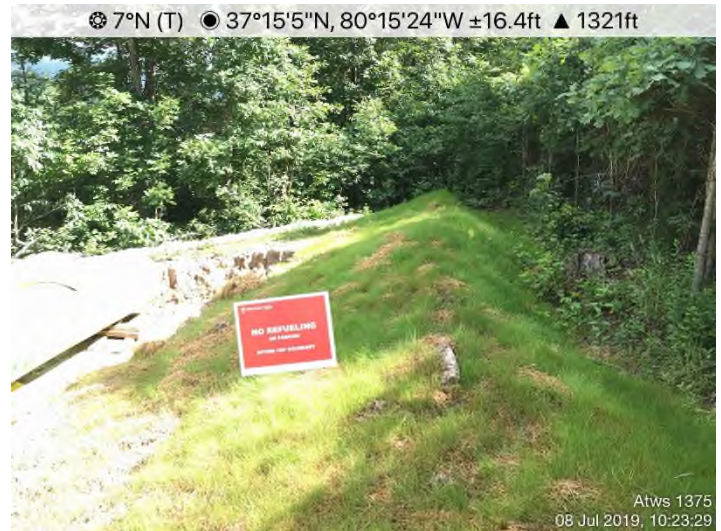
Fig. 12: ATWS 1375 – Looking north from ATWS 1375 towards stream S-OO11. Perimeter diversions berm stabilized with seed and straw.
