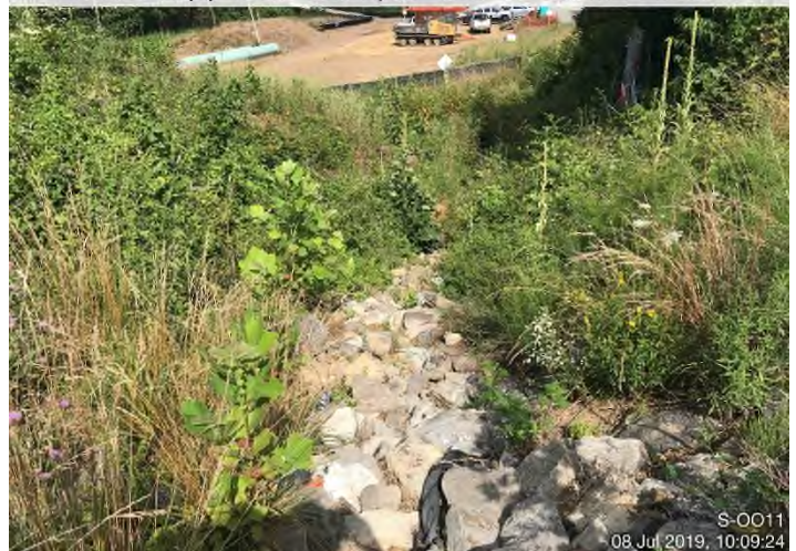
Fig. 8: Stream S-0011 – Riprap outfall channel of S-0011 culvert on west side of Norfolk Western railroad tracks. Riprap appeared to be clean and free of sediment found impacting resource further downstream.
