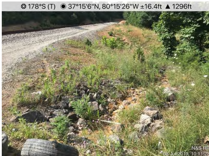
Fig. 11: ATWS 1375 – Looking north from ATWS 1375 towards stream S-OO11. CFS is in good condition. Dormant areas stabilized with seed, straw and fabric.
