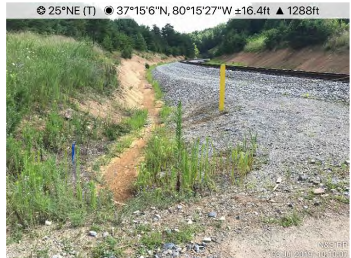
Fig. 12: ATWS 1375 – Looking north from ATWS 1375 towards stream S-OO11. Perimeter diversions berm stabilized with seed and straw.
