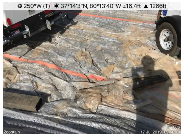
Fig. 4: Pipe Yard 006 – Secondary containment requires maintenance.
