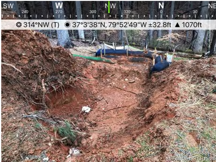
Fig. 7: GAS S-KL39 - Waterbar maintenance needed.
