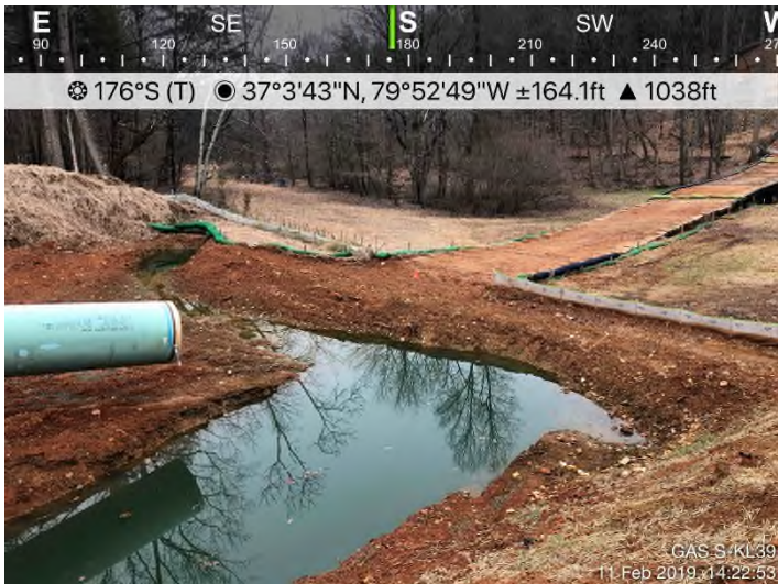
Fig. 7: GAS S-KL39 - Waterbar maintenance needed.
