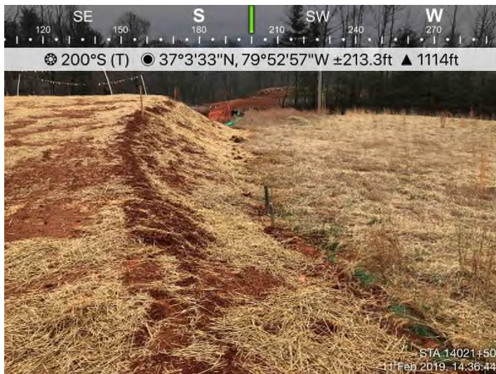
Fig. 3: STA 14021+00 - Perimeter controls overrun.
