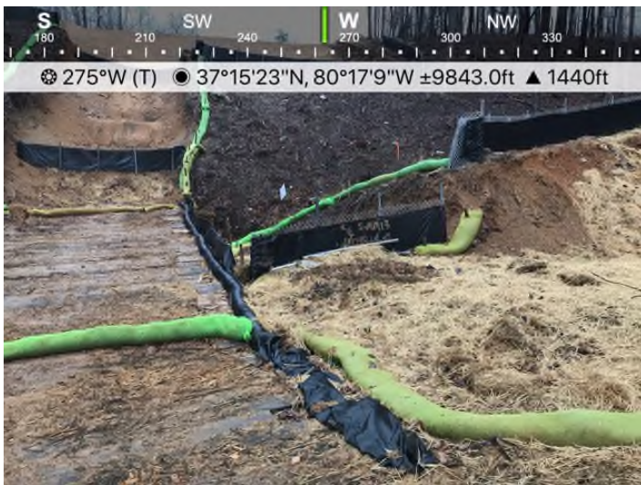
Fig. 3: STA 12098+44 – ECDs installed and maintained around S-MM13.
