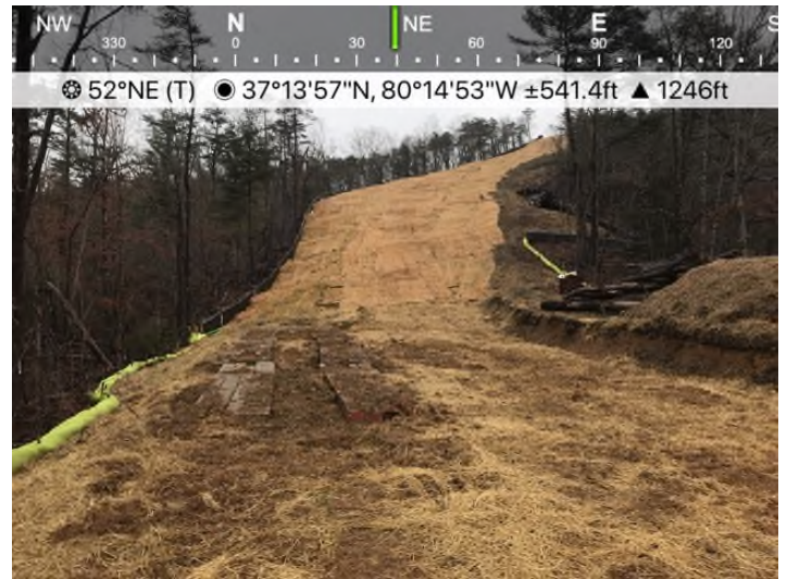
Fig. 4: STA 12098+44 – Temporary crossing for S-MM13 adequately maintained.
