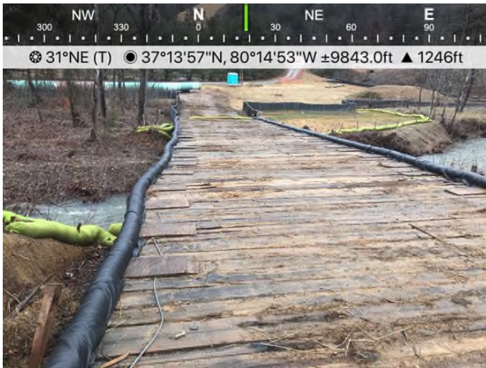
Fig. 3: STA 12098+44 – ECDs installed and maintained around S-MM13.
