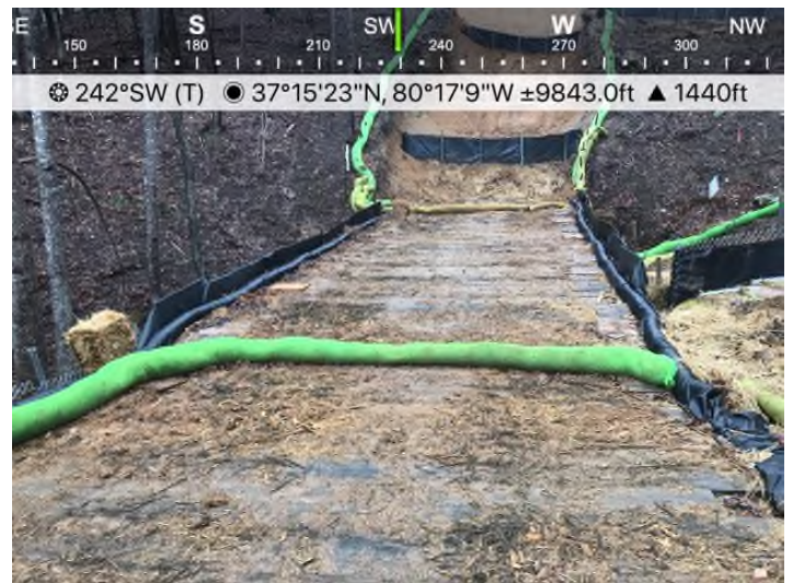
Fig. 4: STA 12098+44 – Temporary crossing for S-MM13 adequately maintained.
