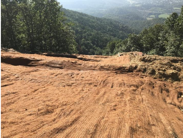
Fig. 1 Near St# 12285+75 blanket matting installed
