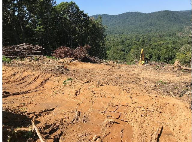
Fig. 2 Near St# 13366+34 waterbar install
