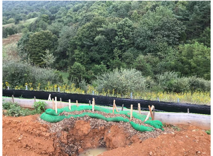
Fig. 4 MP 217 St#11472+00, karsts areas protected with triple stack, P1 & SSF.
