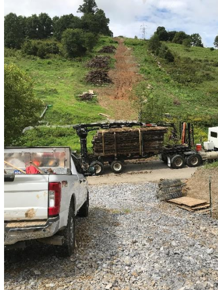
Fig. 2 MP 206 bridge removed at designated stream SA-32
