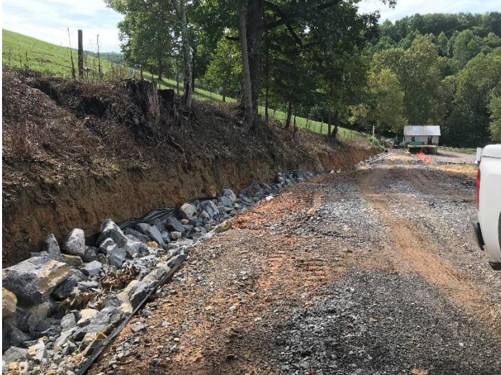
Fig. 1 Access road G-I 234 conveyance channel completed
