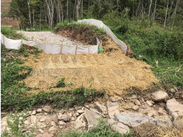
Fig. 3 MP 207 bridge removed at designated stream SY3
