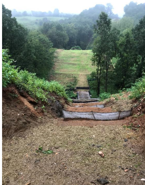
Fig. 4 MP 252.21 St#13317+00 – 13320+00 blanket matting has been installed.
