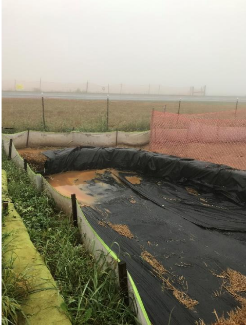
Fig. 1 MP 246.47 St#13014+00 dewatering structure in place
