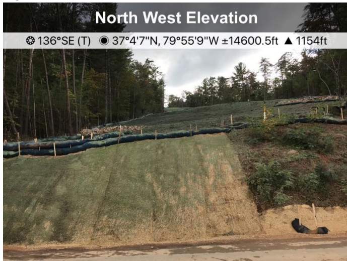
Fig. 1 At Cahas Rd intersection, matting has been installed with ECD's.
