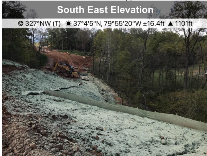
Fig. 1 At St#13819 stabilization has been applied.
