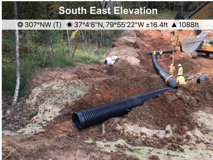
Fig. 3 At St#13817+10 clean water pipe install.
