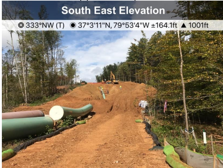
Fig. 1 At St# 13998+10 the pipe has been placed in trench.
