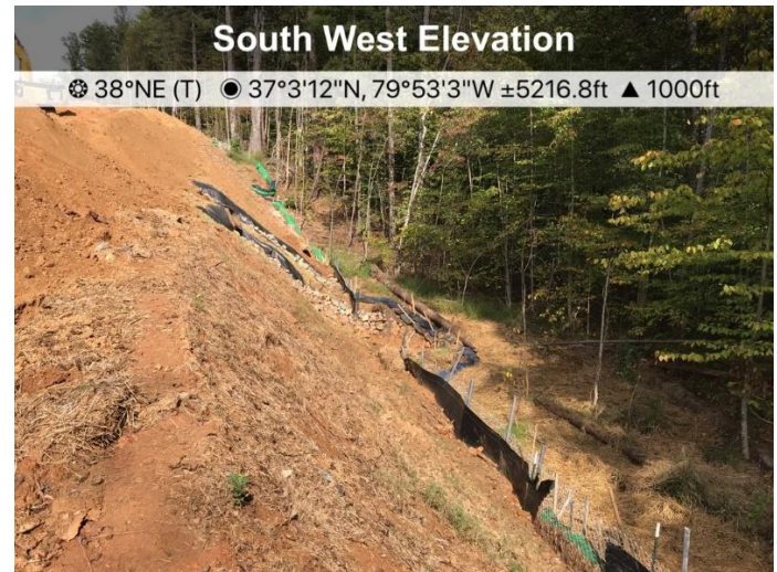
Fig. 2 At St#13998+10 ECD's are in place below slope
