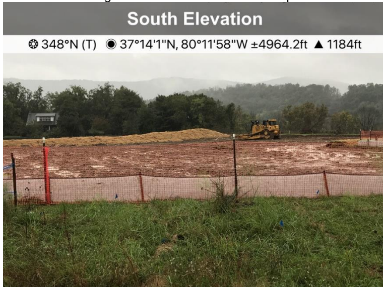
Fig. 3 Route 11 crossing near St#12453 ECD's are in place.
