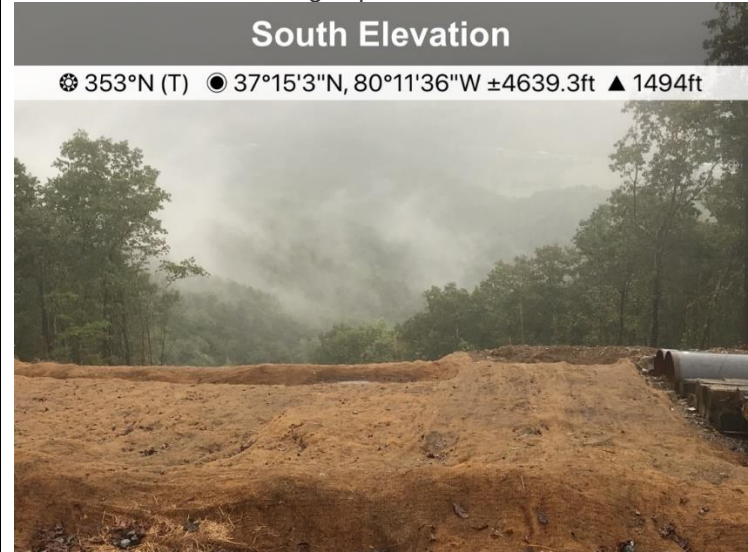
Fig. 2 MP 232 St#12283 matting in place at Reese Mtn.
