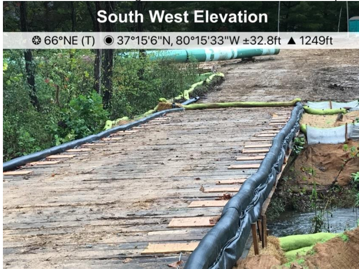
Fig. 1 MP 230 St#12192 designated stream SC21 ECD's are in place.
