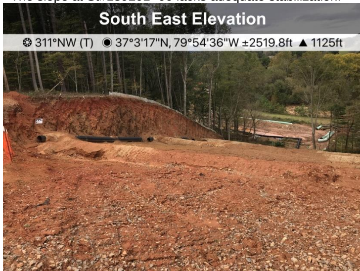
Fig. 7 The slope at St#139201+00 lacks adequate stabilization.
