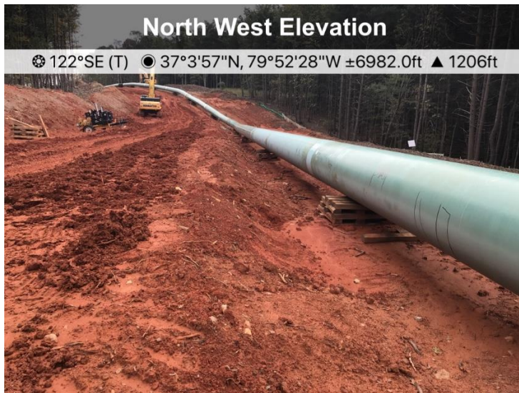
Fig. 7 The slope at St#139201+00 lacks adequate stabilization.
