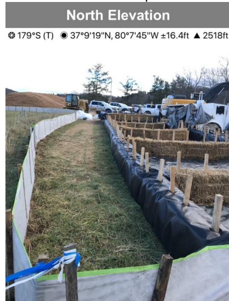
Fig. 2 Dewatering structure in place and functioning at the Bottoms Creek bore pit.
