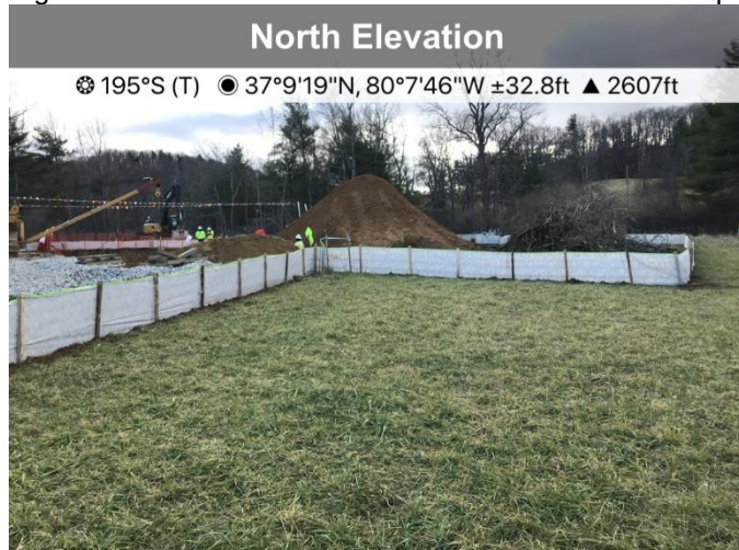
Fig. 3 Work within the LOD of the Bottoms Creek bore pit.
