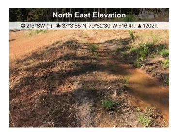
Fig. 6 St14063 stabilization matting requires repair
