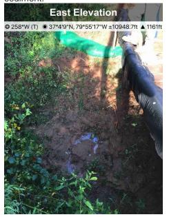
Fig. 2 St13805 P1 is down, repair or replace with adequate control
