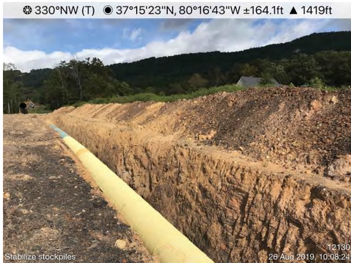
Fig. 3: STA 12130+00 to 12187+00 – Stockpile stabilization needed.
