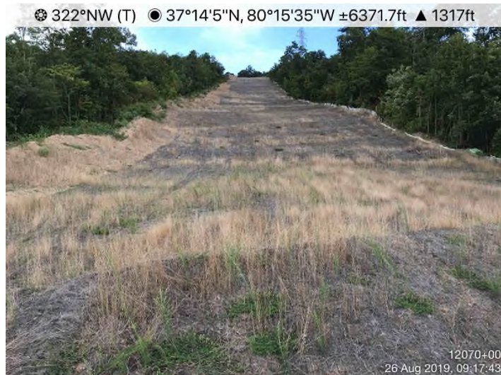
Fig. 3: STA 12130+00 to 12187+00 – Stockpile stabilization needed.
