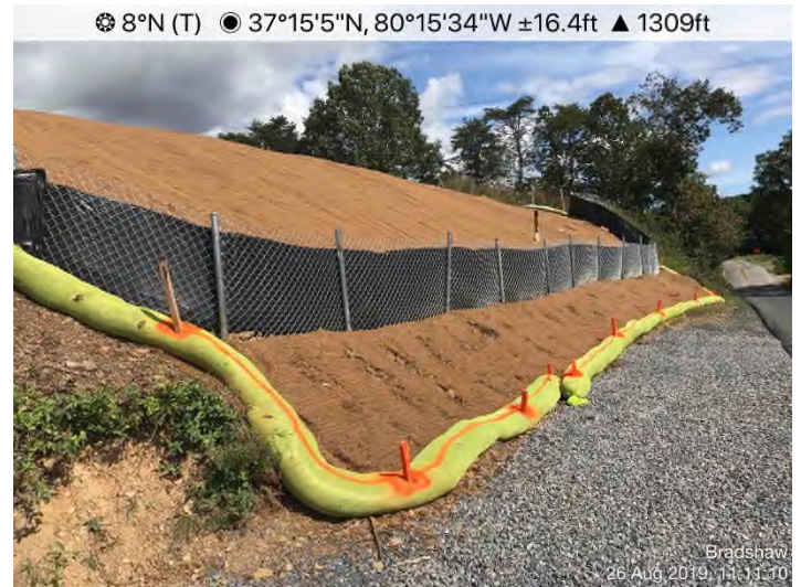
Fig. 4: STA 12190+85 – Bradshaw Road crossing. Controls in place. Stabilized with erosion fabric and seed.
