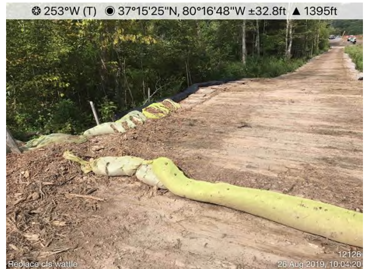
Fig. 4: STA 12190+85 – Bradshaw Road crossing. Controls in place. Stabilized with erosion fabric and seed.
