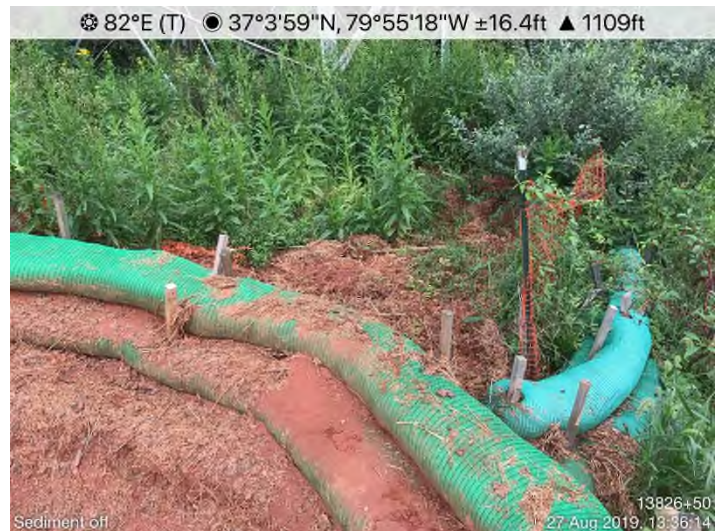
Fig. 8: STA 13826+50 – Sediment off ROW.
