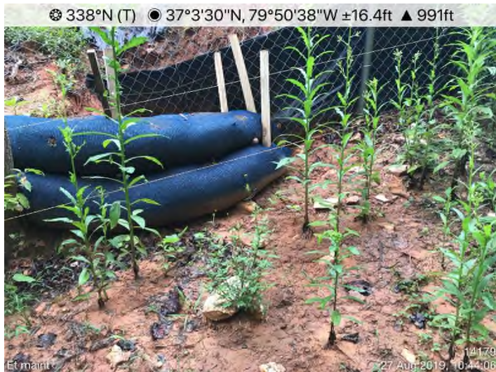
Fig. 7: STA 14199+00 – CFS maintenance needed.
