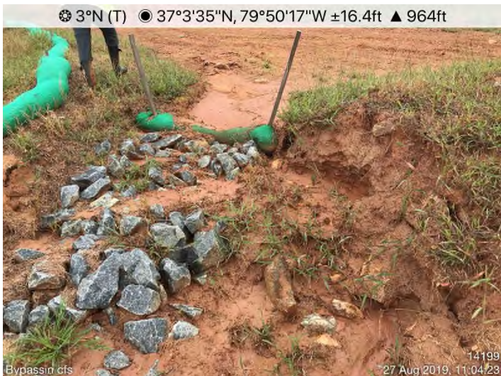
Fig. 7: STA 14199+00 – CFS maintenance needed.
