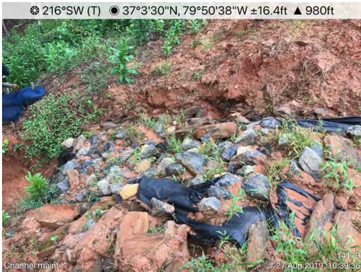
Fig. 3: STA 14179+00 – Rock swale maintenance needed.
