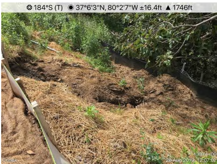
Fig. 3: STA 13374+00 – Repair and stabilize slope.
