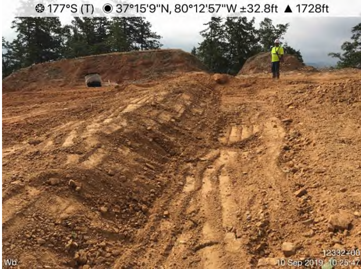
Fig. 7: STA 12321+00 to 12356+00 – Waterbars do not have positive drainage to end treatments.
