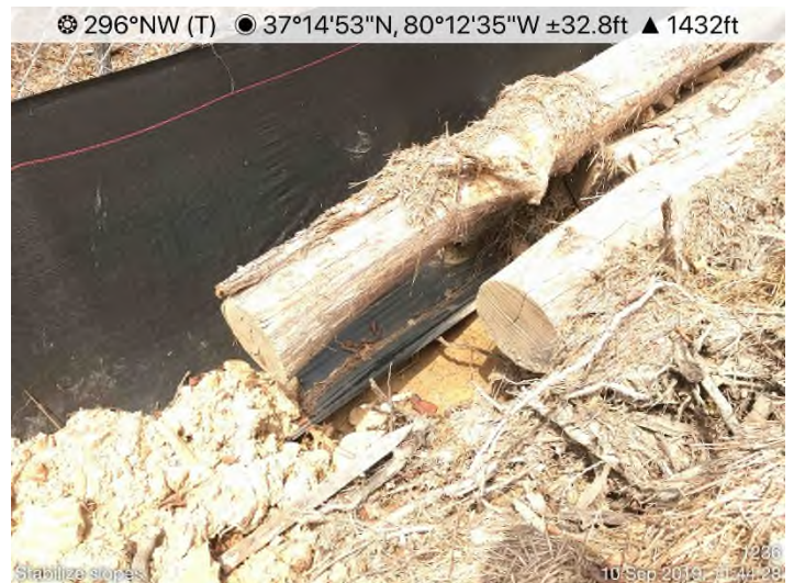
Fig. 4: STA 12361+10 – SSF undermined.
