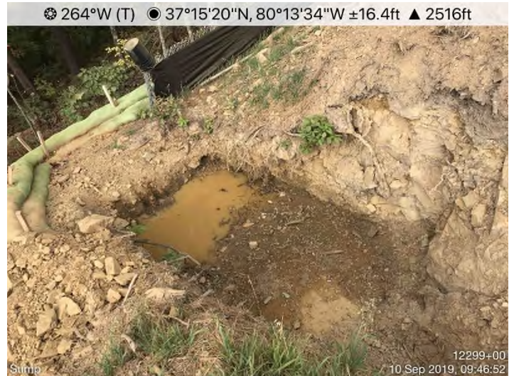
Fig. 4: STA 12361+10 – SSF undermined.
