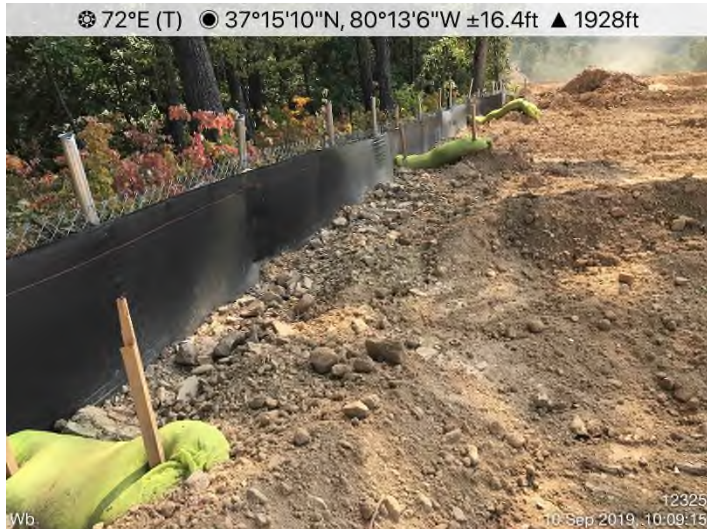
Fig. 7: STA 12321+00 to 12356+00 – Waterbars do not have positive drainage to end treatments.
