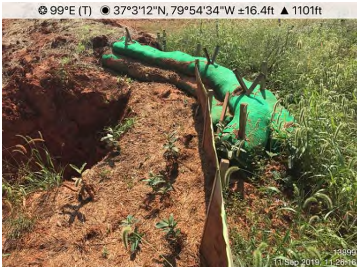
Fig. 3: STA 13898+00 – Discharge bypassing end-treatment.
