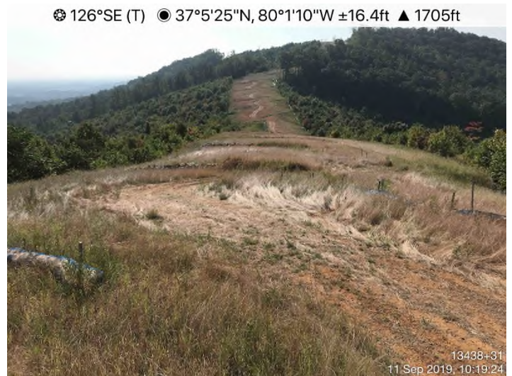
Fig. 4: STA 13899+00 – Inadequate stabilization outside of travel lane.
