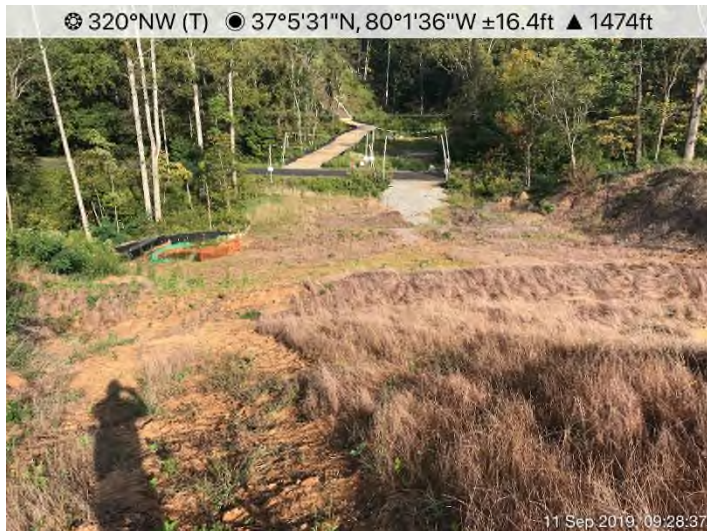
Fig. 3: STA 13898+00 – Discharge bypassing end-treatment.
