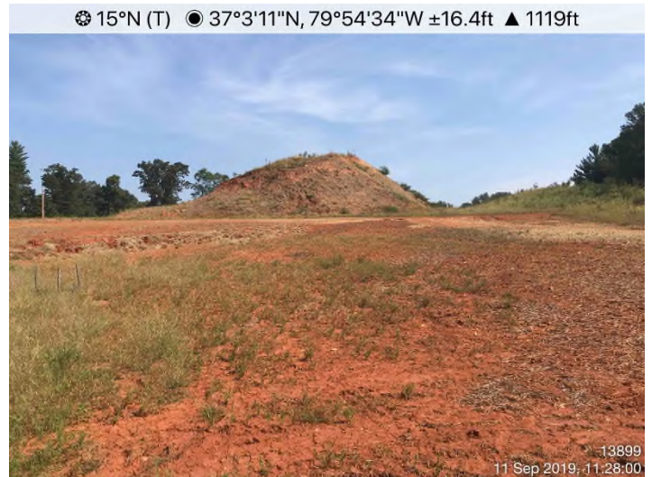
Fig. 4: STA 13899+00 – Inadequate stabilization outside of travel lane.
