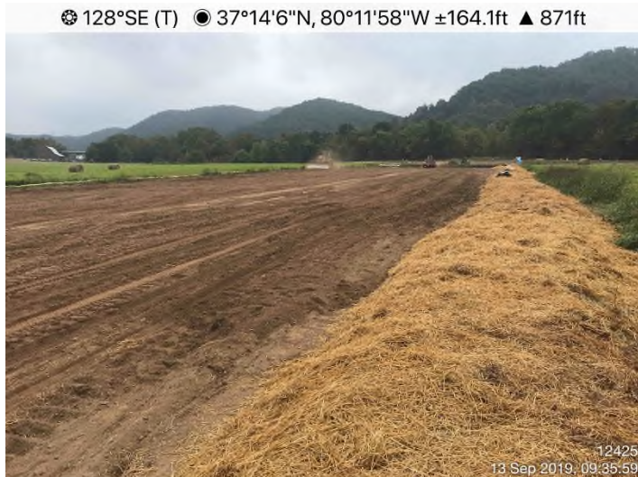
Fig. 3: STA 12433+00 – Stabilization in progress in ATWS 725.
