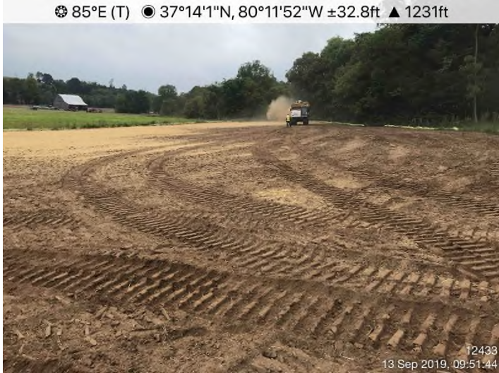
Fig. 3: STA 12433+00 – Stabilization in progress in ATWS 725.
