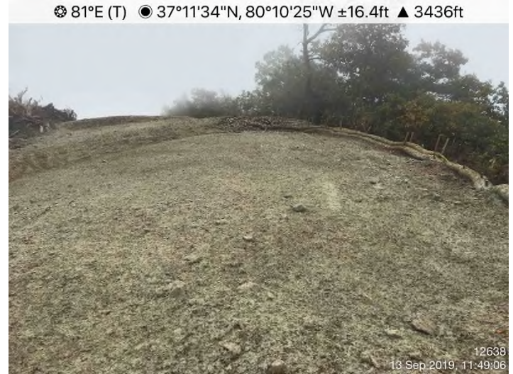
Fig. 4: STA 12638+00 – Controls in place. Area stabilized with hydro-mulch and erosion blanket.
