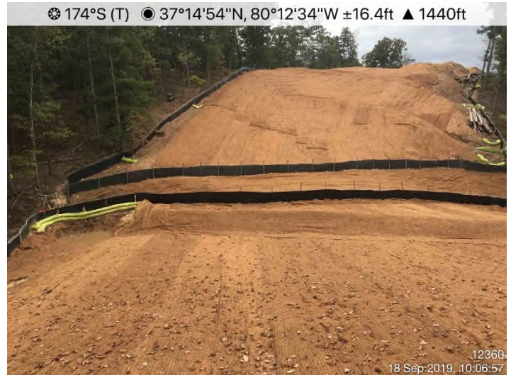
Fig. 4: STA 12637+17 – Controls in place. Area stabilized with seed, Proganics and Flexterra
