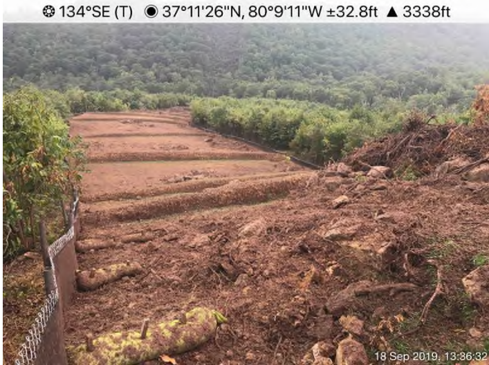
Fig. 3: STA 12705+00 – Controls in place. Area stabilized with seed, Proganics and Flexterra
