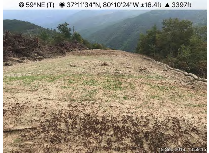
Fig. 4: STA 12637+17 – Controls in place. Area stabilized with seed, Proganics and Flexterra
