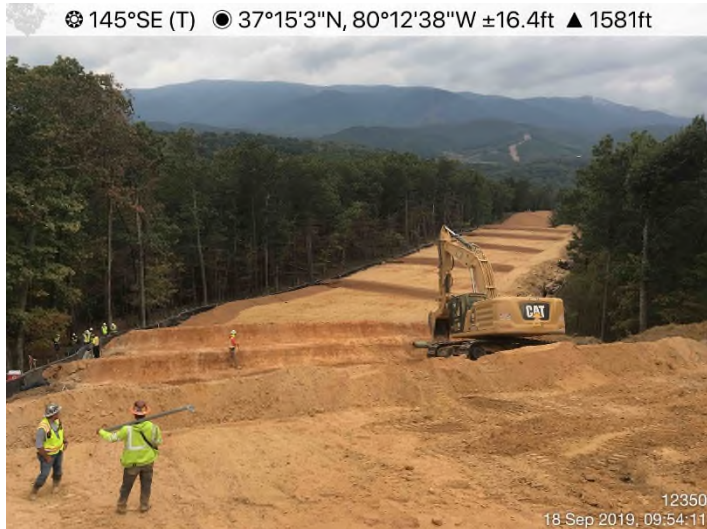
Fig. 3: STA 12705+00 – Controls in place. Area stabilized with seed, Proganics and Flexterra
