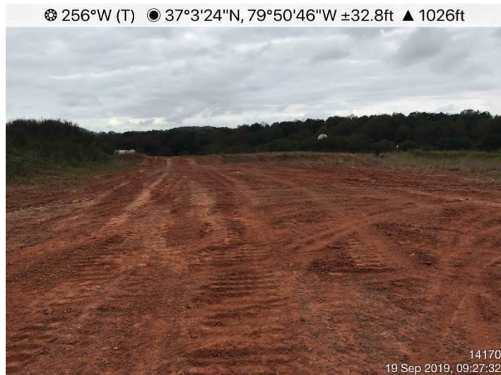
Fig. 3: STA 14091+00 – Controls in place. Area stabilized with seed and Earth Guard Edge.
