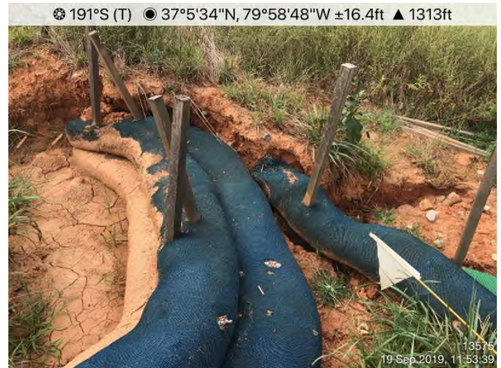
Fig. 4: STA 13575+00 – CFS undermined.
