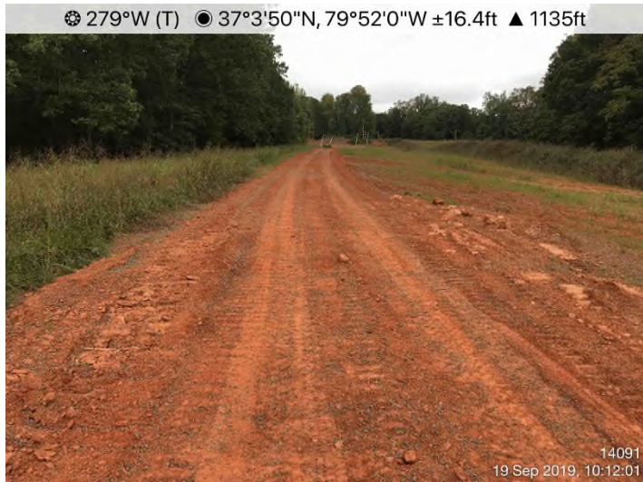
Fig. 3: STA 14091+00 – Controls in place. Area stabilized with seed and Earth Guard Edge.
