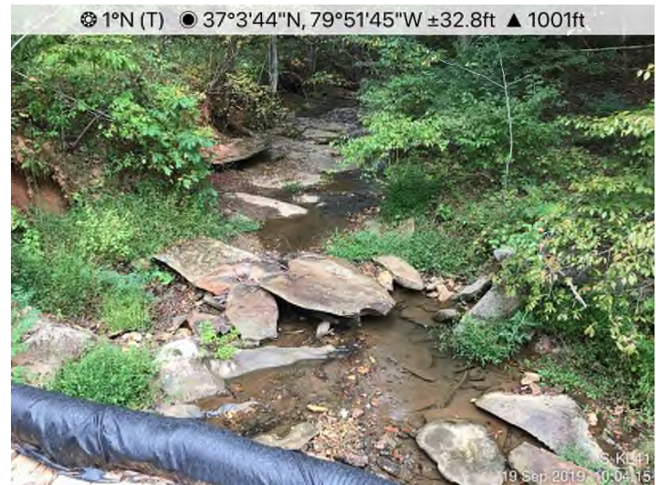
Fig. 4: STA 13575+00 – CFS undermined.
