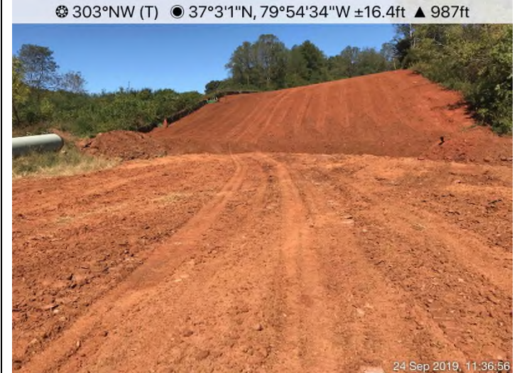
Fig. 8: STA 13908+00 – Final grading in progress. Spreading topsoil and re-establishing grade to existing contours.
