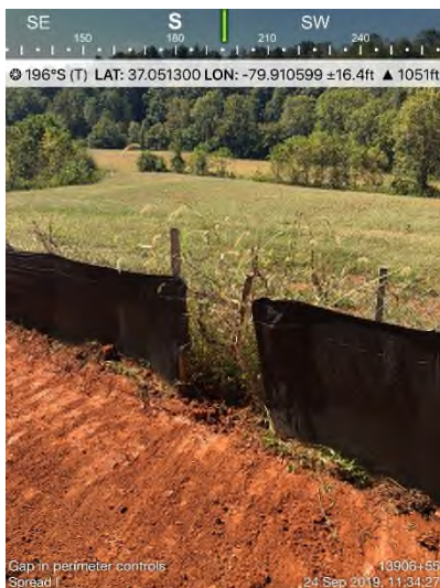
Fig. 7: STA 13906+55 – SSF maintenance need.
