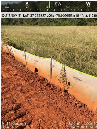
Fig. 7: STA 13906+55 – SSF maintenance need.
