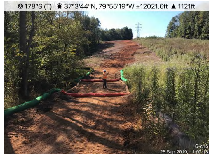
Fig. 4: STA 13745+00 – Controls in place. Final grading in progress. Actively hydro-seeding in this area.
