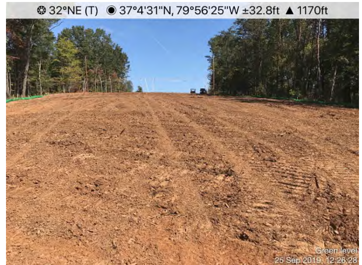
Fig. 4: STA 13745+00 – Controls in place. Final grading in progress. Actively hydro-seeding in this area.
