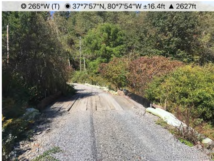
Fig. 3: MVP-RO-288 – Stream S-Q20 crossing. Controls in place and functioning properly.
