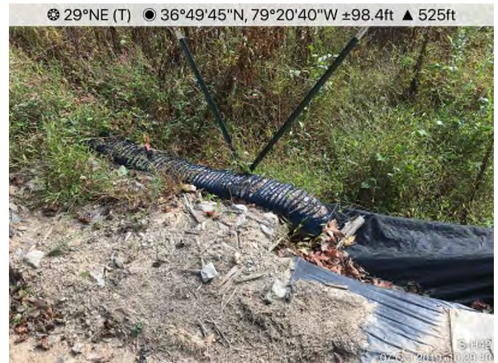
Fig. 4: STA 15970+00 – CFS maintenance needed.
