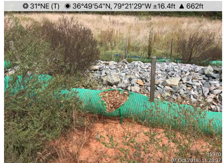
Fig. 4: STA 15970+00 – CFS maintenance needed.
