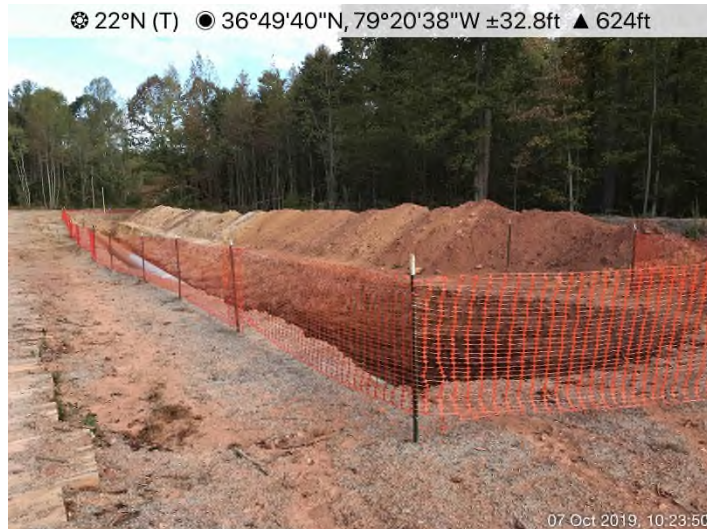
Fig. 3: Stream S-001 – Stabilization needed on both sides of stream crossing.
