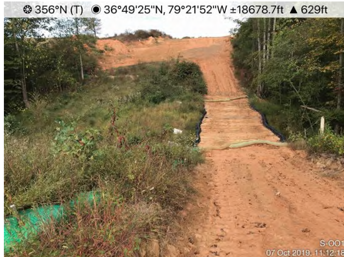
Fig. 3: Stream S-001 – Stabilization needed on both sides of stream crossing.
