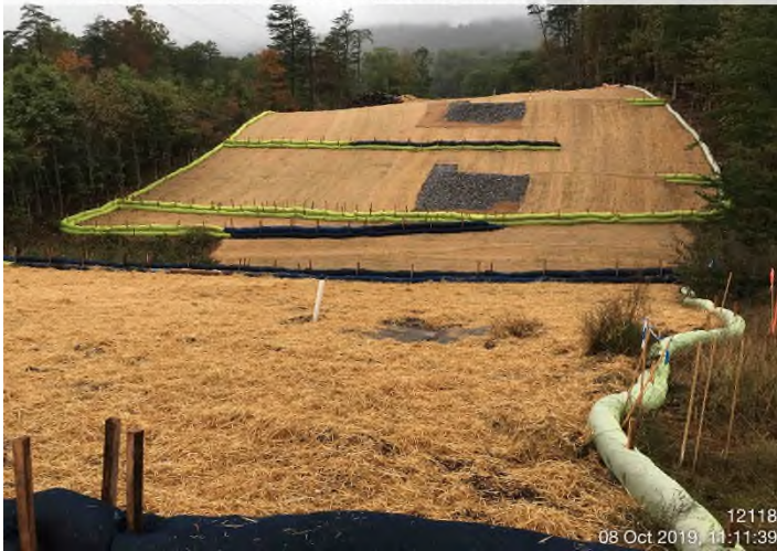
Fig. 3: STA 12117+62 – Controls in place. Area stabilized with straw and erosion matting.
