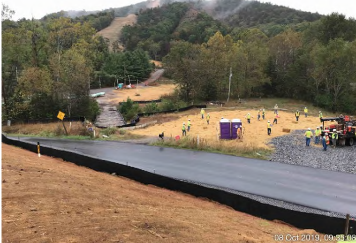
Fig. 3: STA 12117+62 – Controls in place. Area stabilized with straw and erosion matting.
