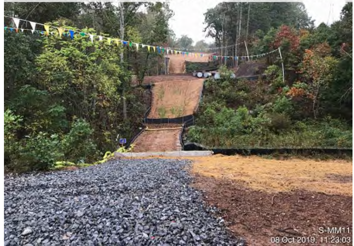
Fig. 4: Stream S-MM11 – Controls in place. Area stabilized with straw and erosion matting.
