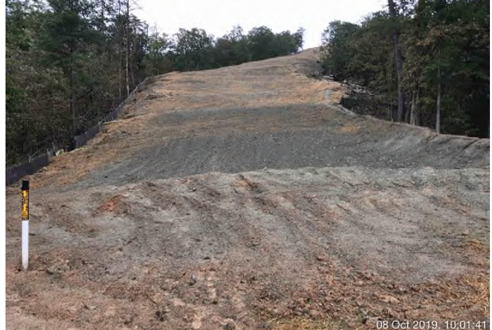
Fig. 4: Stream S-MM11 – Controls in place. Area stabilized with straw and erosion matting.
