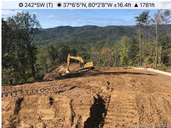
Fig. 3: STA 13370+00 – Controls in place. Area actively being graded back to subgrade.
