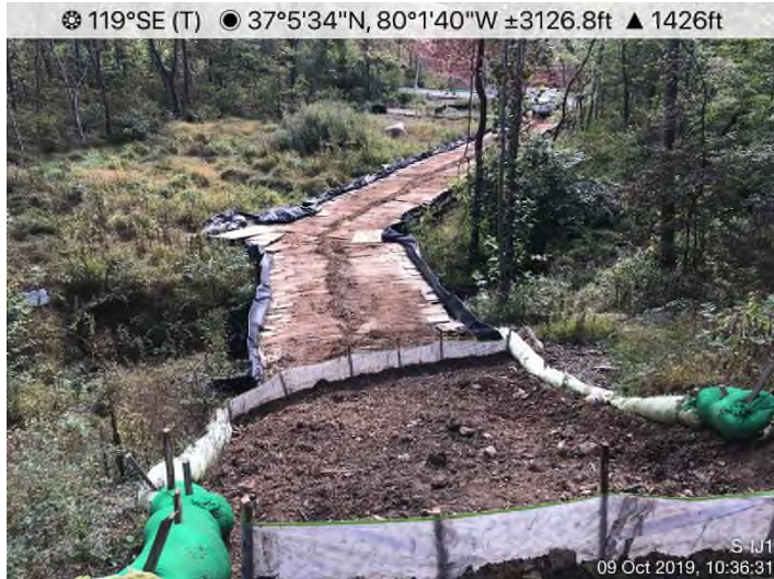
Fig. 3: STA 13370+00 – Controls in place. Area actively being graded back to subgrade.
