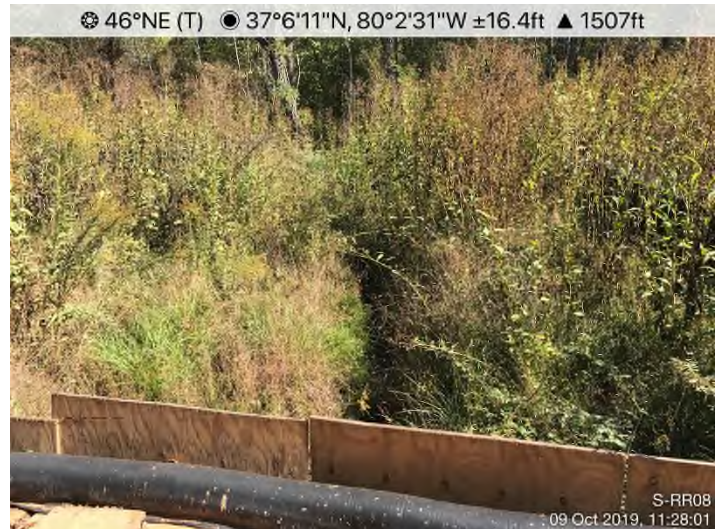
Fig. 4: Stream S-RR08 – Controls in place at stream crossing and functioning properly.
