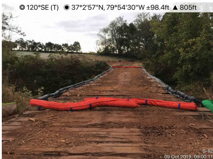
Fig. 3: Stream S-II2 – Controls in place and functioning properly at stream crossing.
