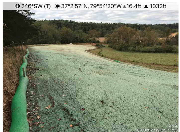
Fig. 4: STA 13925+00 – Controls in place. Area stabilized with hydro-mulch.
