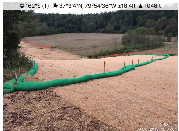
Fig. 4: STA 13925+00 – Controls in place. Area stabilized with hydro-mulch.
