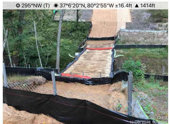
Fig. 4: STA 13300+00 – Controls in place. Area actively being worked to final restoration.
