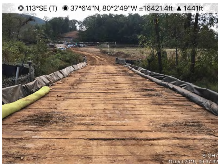
Fig. 3: Stream S-GH7 – Controls in place and functioning properly.
