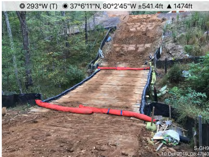
Fig. 3: Stream S-GH7 – Controls in place and functioning properly.
