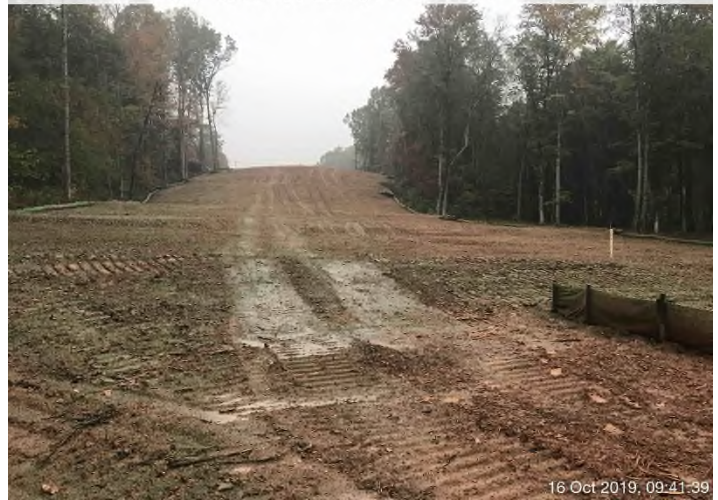
Fig. 4: STA 14656+37 – Controls in place and area stabilized with hydraulic mulch.
