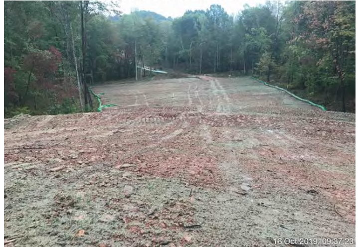
Fig. 4: STA 14656+37 – Controls in place and area stabilized with hydraulic mulch.
