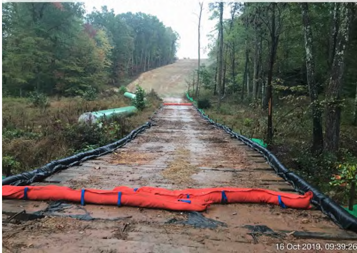
Fig. 3: Stream S-H38 – Controls in place and functioning properly.
