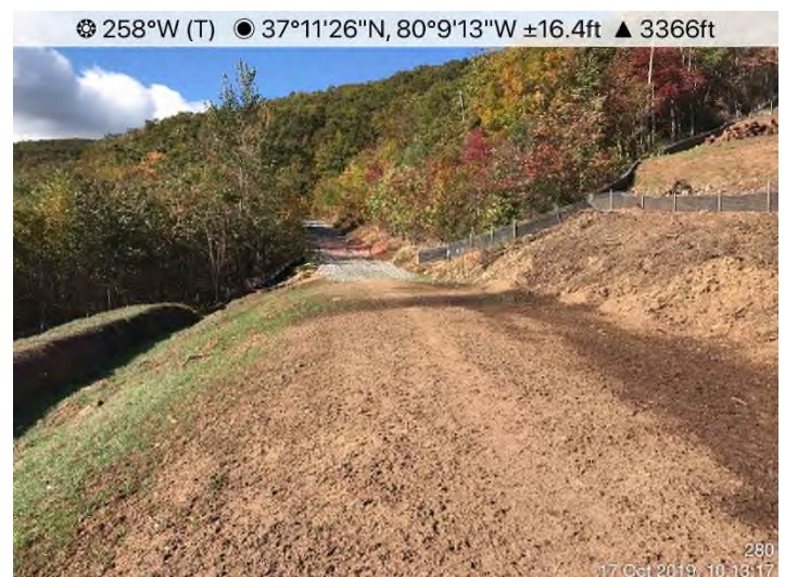
Fig. 4: MVP-RO-288 – Controls in place. Area stabilized with Proganics soil media and hydraulic mulch.
