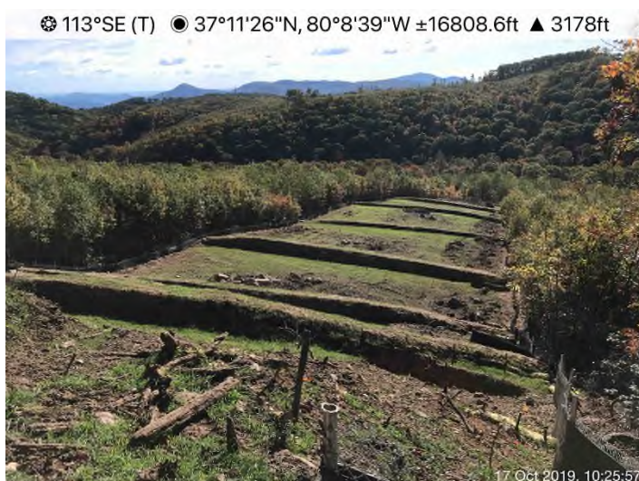
Fig. 3: STA 12703+08 – Controls in place. Area stabilized with Proganics soil media and hydraulic mulch.
