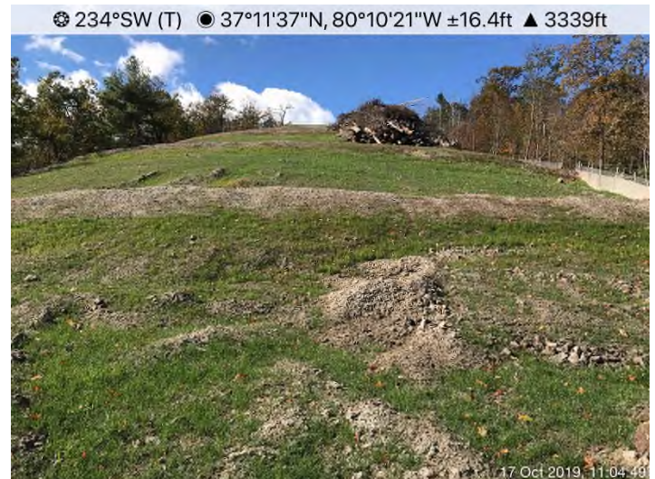
Fig. 4: MVP-RO-288 – Controls in place. Area stabilized with Proganics soil media and hydraulic mulch.
