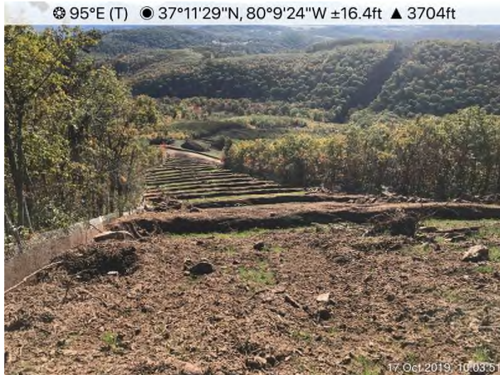
Fig. 3: STA 12703+08 – Controls in place. Area stabilized with Proganics soil media and hydraulic mulch.
