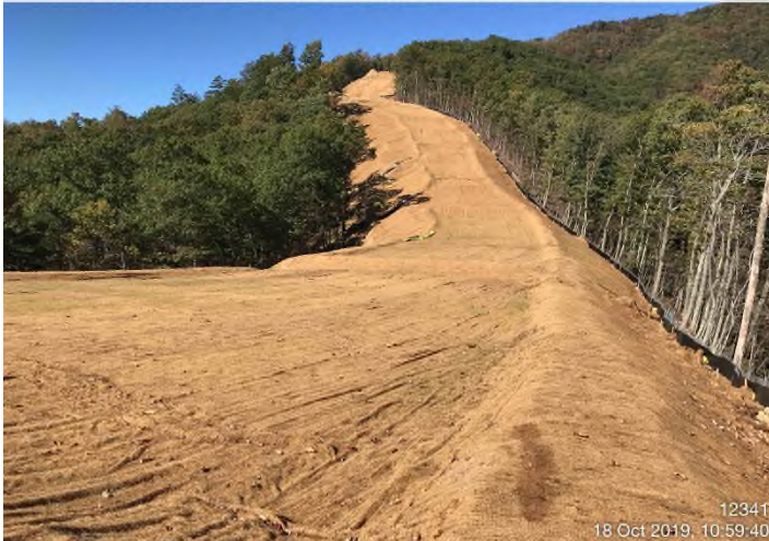
Fig. 3: STA 12341+00 – Controls in place and area stabilized with matting and straw.
