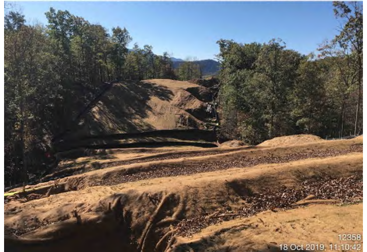
Fig. 4: STA 12358+00 – Controls in place and area stabilized with matting and straw.
