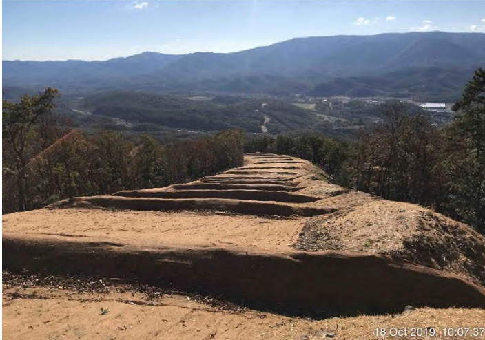
Fig. 3: STA 12341+00 – Controls in place and area stabilized with matting and straw.
