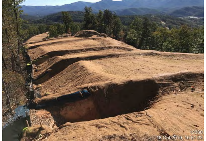
Fig. 4: STA 12358+00 – Controls in place and area stabilized with matting and straw.
