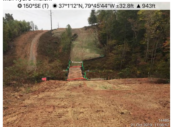
Fig. 4: STA 14485+00 – Controls in place. Area stabilized with hydro-mulch.
