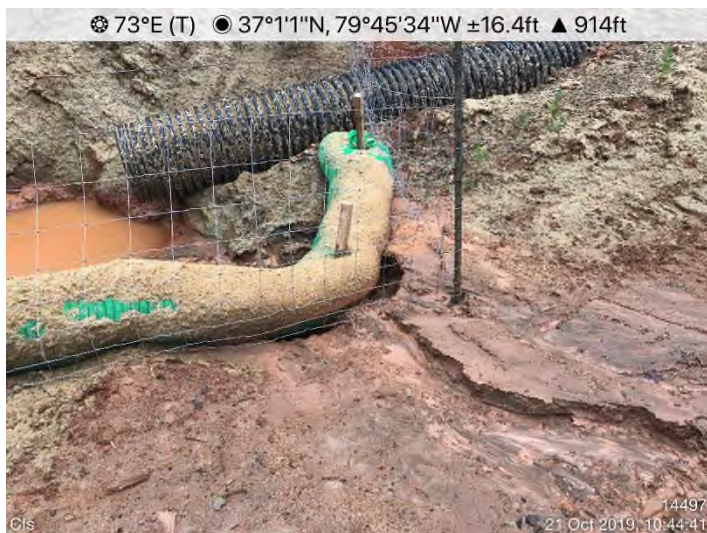
Fig. 3: STA 14497+00 – CFS undermined.
