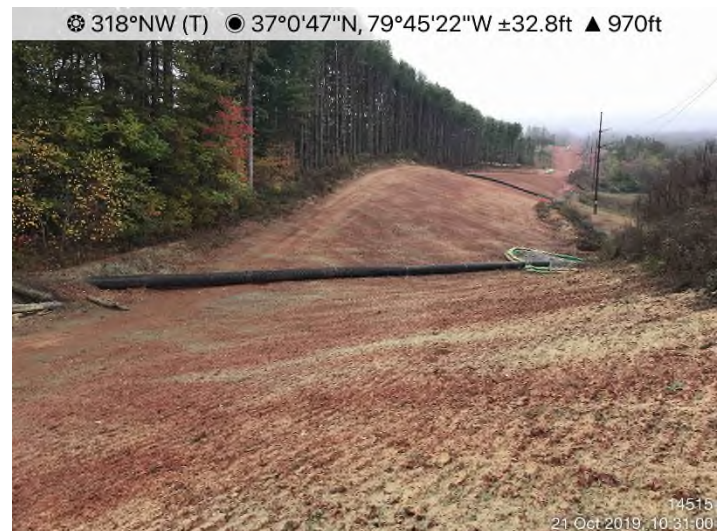
Fig. 4: STA 14485+00 – Controls in place. Area stabilized with hydro-mulch.
