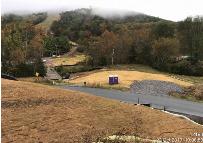
Fig. 3: STA 12117+62 – Controls in place. Area stabilized.
