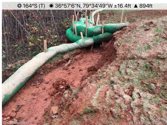
Fig. 15: STA 15128+65 – CFS undermined. Maintenance needed.
