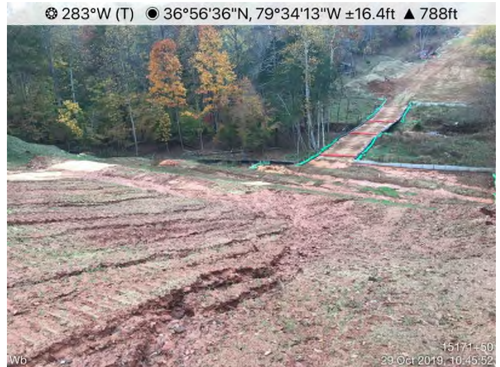
Fig. 4: STA 15169+58 – CFS overtopped. Maintenance needed.
