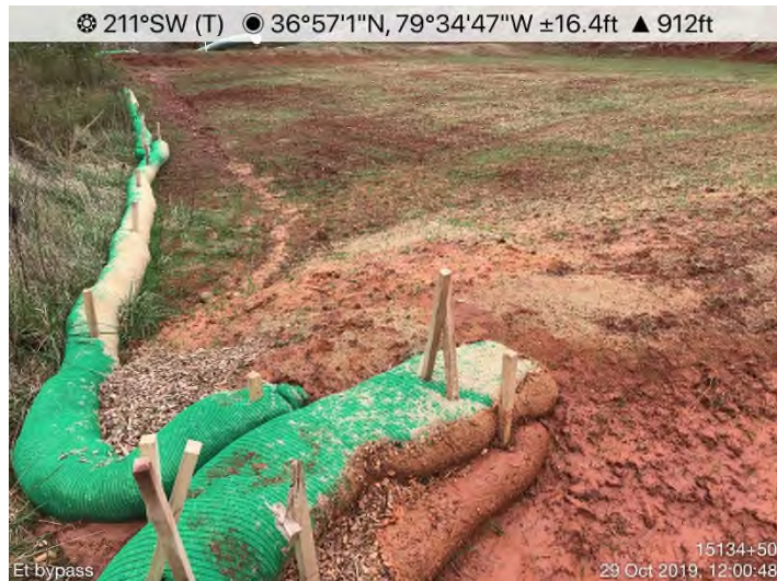
Fig. 15: STA 15128+65 – CFS undermined. Maintenance needed.
