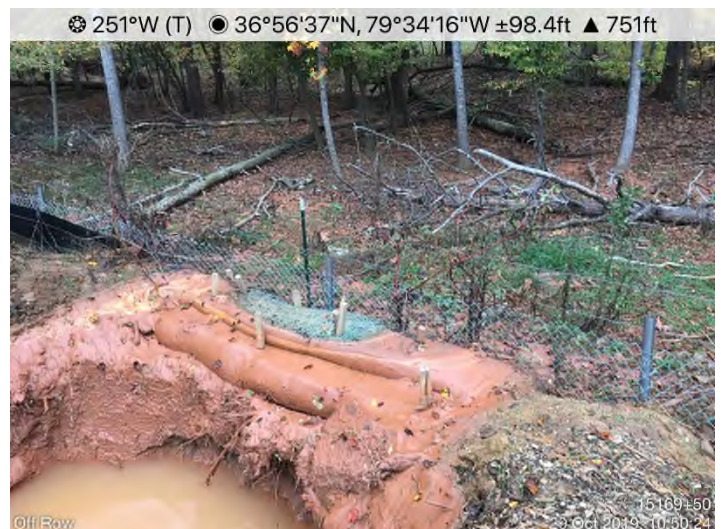
Fig. 4: STA 15169+58 – CFS overtopped. Maintenance needed.
