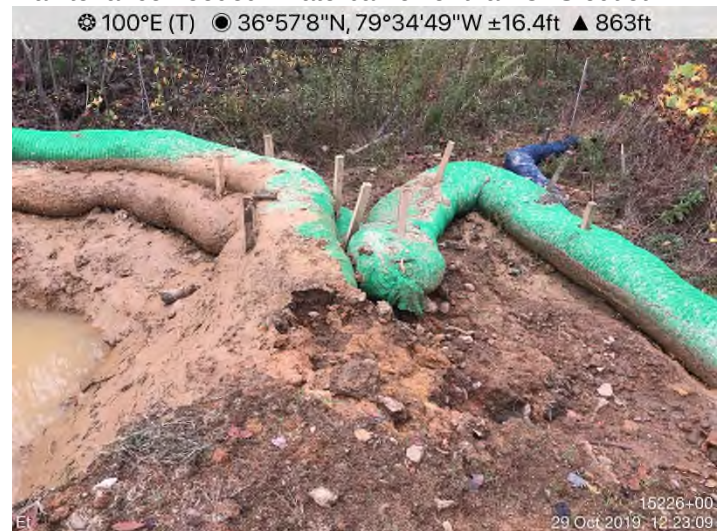
Fig. 20: STA 15126+00 – CFS end-treatment bypassed. Maintenance needed. Waterbar lower than CFS outlet.
