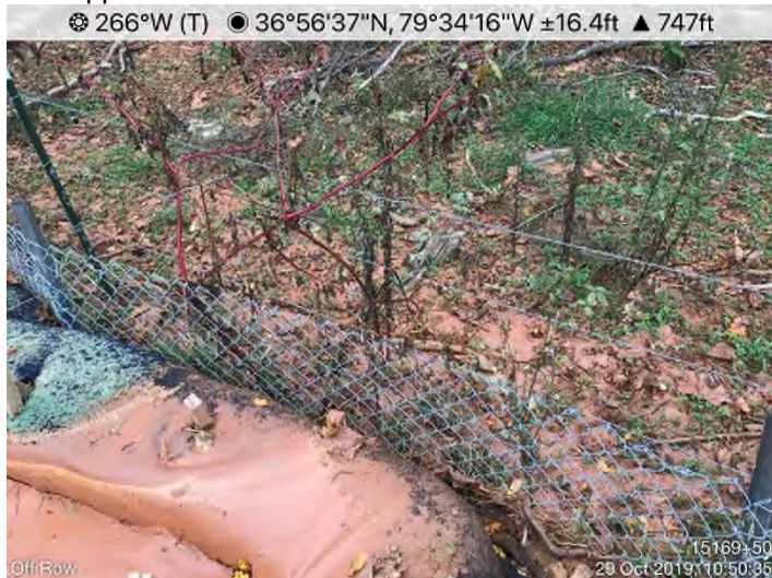
Fig. 3: STA 15169+58 – Sediment off ROW. Controls overtopped.
