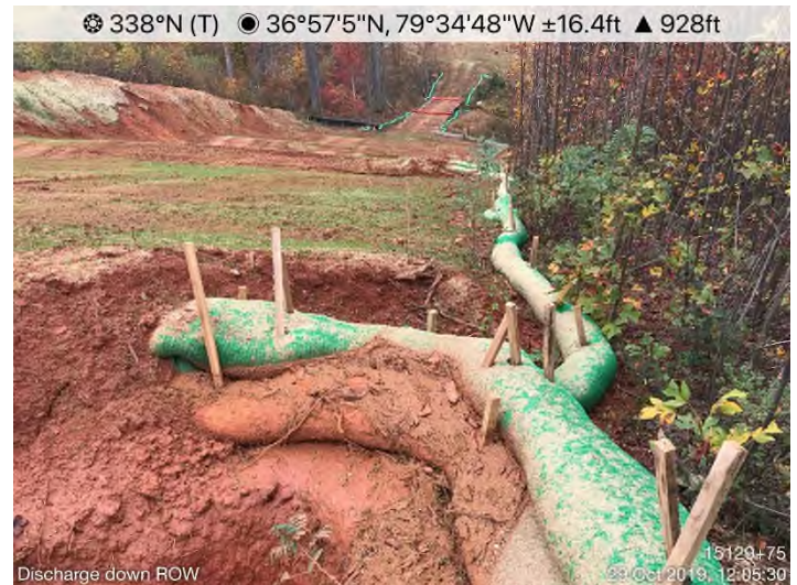
Fig. 16: STA 15128+40 – Sediment off ROW due to upslope control failure and incorrect installation of waterbar end treatments.
