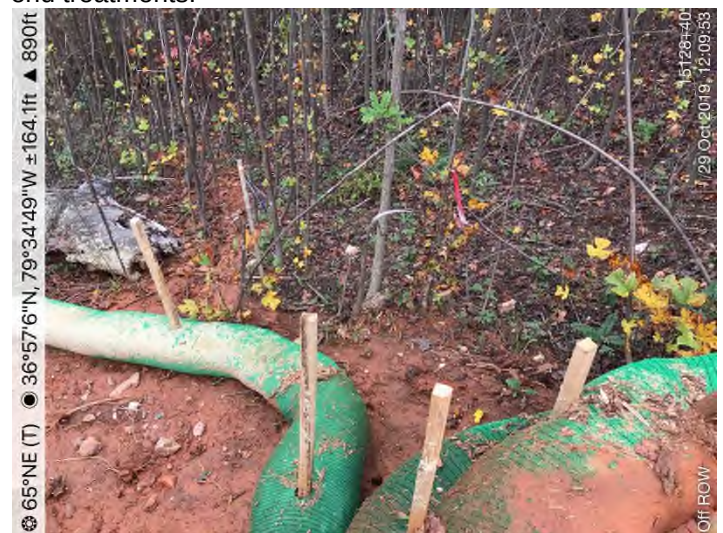
Fig. 16: STA 15128+40 – Sediment off ROW due to upslope control failure and incorrect installation of waterbar end treatments.
