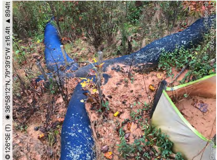
Fig. 16: STA 14888+75 – Stabilize slope/repair erosion adjacent to S-AB8.
