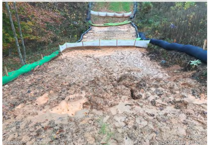
Fig. 16: STA 14888+75 – Stabilize slope/repair erosion adjacent to S-AB8.
