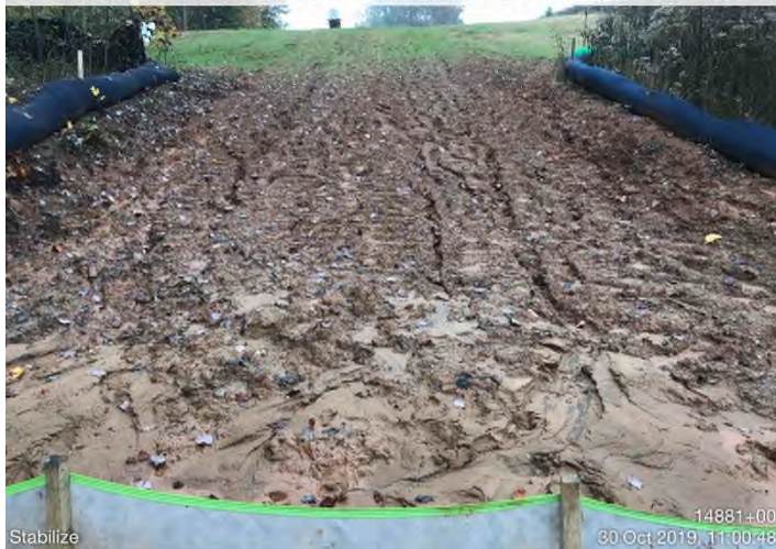
Fig. 9: STA 14881+00 – Stabilize slope/repair erosion adjacent to S-CD8.
