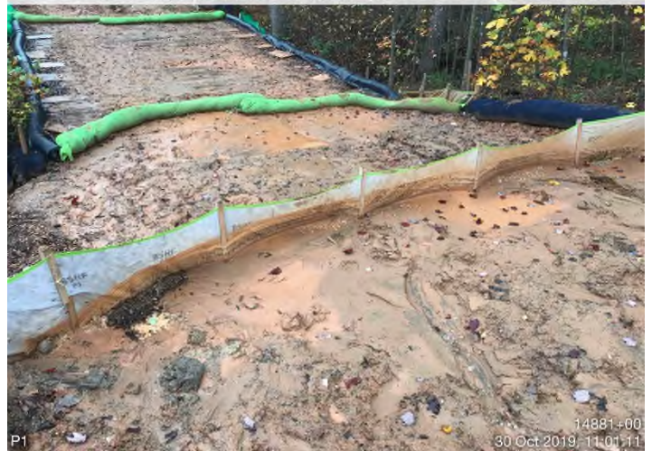
Fig. 12: STA 14888+10 – Sump maintenance needed.
