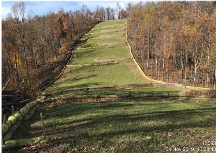
Fig. 3: STA 13093+00 – Controls in place and functioning properly. Area stabilized with Proganics and flexterra.
