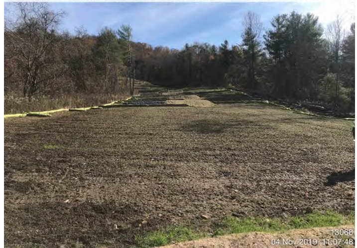
Fig. 4: STA 13068+00 – Controls in place and functioning properly. Area stabilized with Proganics and flexterra.
