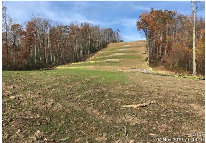
Fig. 4: STA 13068+00 – Controls in place and functioning properly. Area stabilized with Proganics and flexterra.
