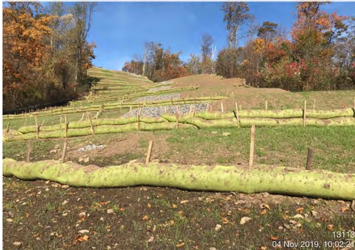
Fig. 3: STA 13093+00 – Controls in place and functioning properly. Area stabilized with Proganics and flexterra.
