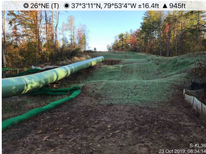
Fig. 3: Stream S-E28 – Controls in place along Teels Creek.
