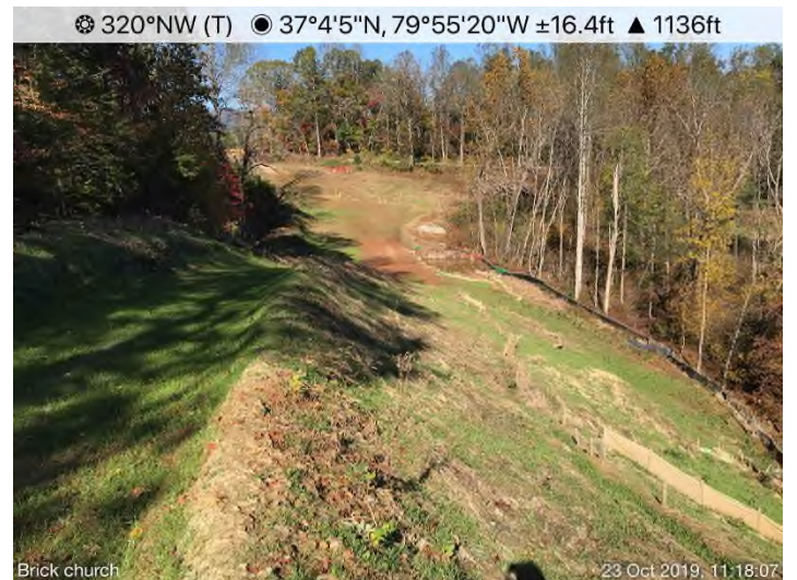
Fig. 4: STA 13820+00 – Controls in place. Area stabilized.
