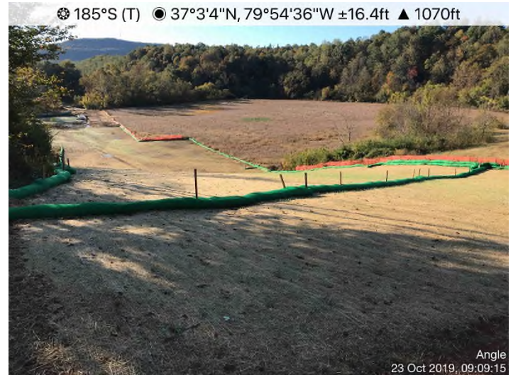
Fig. 4: STA 13820+00 – Controls in place. Area stabilized.
