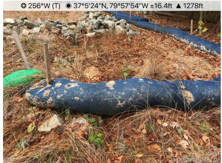
Fig. 2: STA 13631+00 – CFS undermined.
