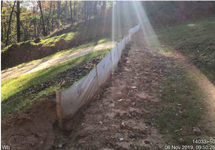
Fig. 3: STA 14033+50 – Waterbar maintenance needed.
