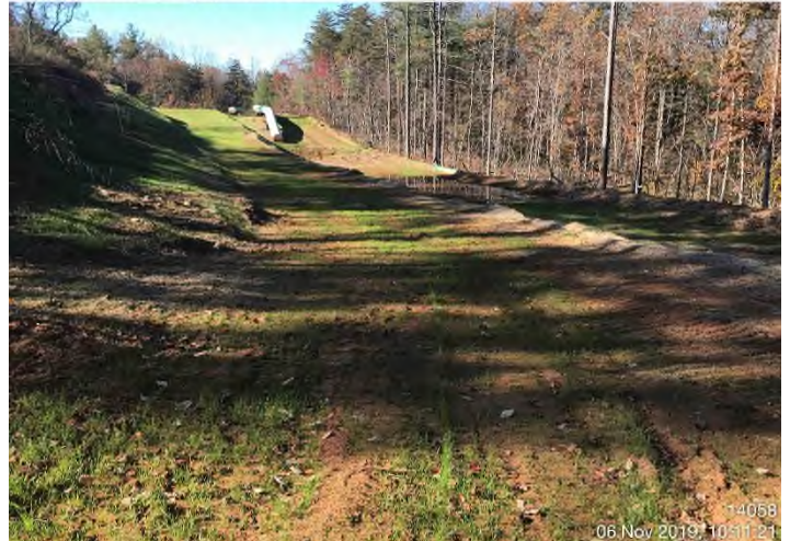
Fig. 4: STA 14058+00 – Controls in place and functioning properly. Area adequately stabilized.
