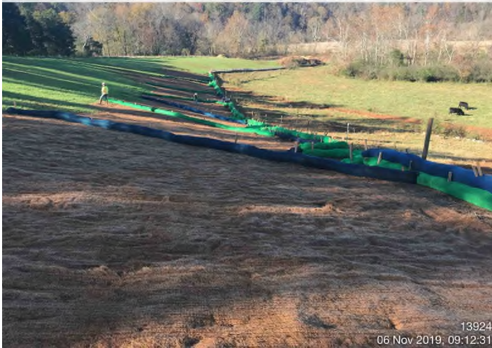
Fig. 3: STA 14033+50 – Waterbar maintenance needed.
