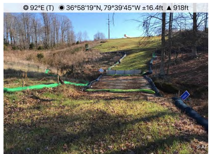
Fig. 4: STA 14854+00 – Controls in place and functioning along stream S-A7. Area stabilized with vegetative cover.
