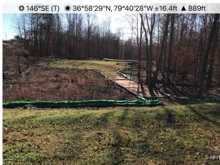
Fig. 3: STA 14815+50 – Controls in place and functioning along stream S-HH1. Area stabilized with vegetative cover.
