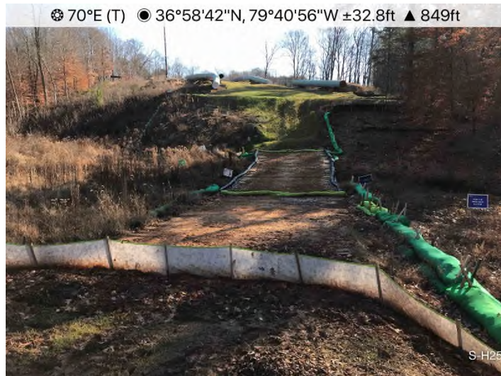
Fig. 3: STA 14815+50 – Controls in place and functioning along stream S-HH1. Area stabilized with vegetative cover.
