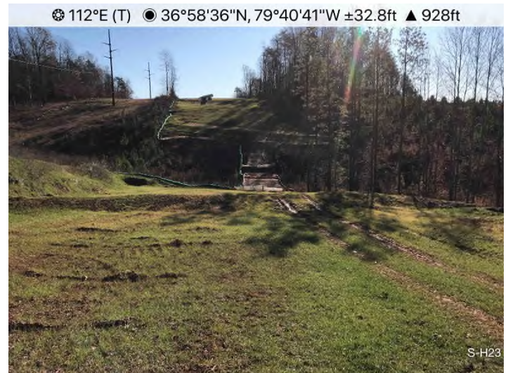
Fig. 4: STA 14854+00 – Controls in place and functioning along stream S-A7. Area stabilized with vegetative cover.
